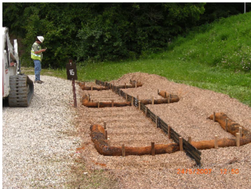
Figure 21. Post-construction Reactive Filter Barrier Installation on the North Kinder Range at Fort Leavenworth, KS.
