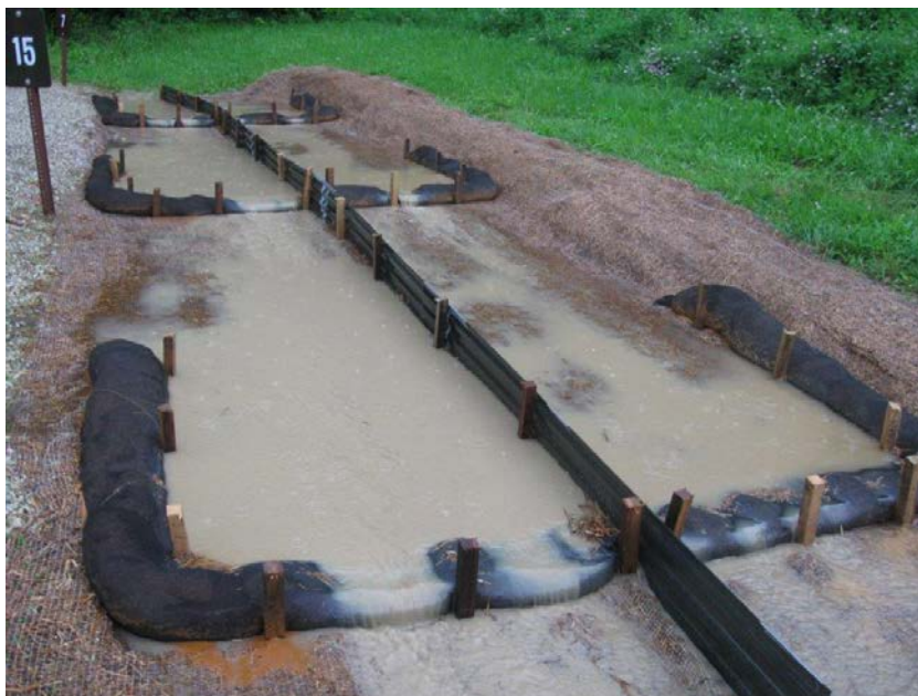
Figure 25. Reactive Filter Barriers on the North Kinder Range during Heavy Rain on 4 June 2015.
