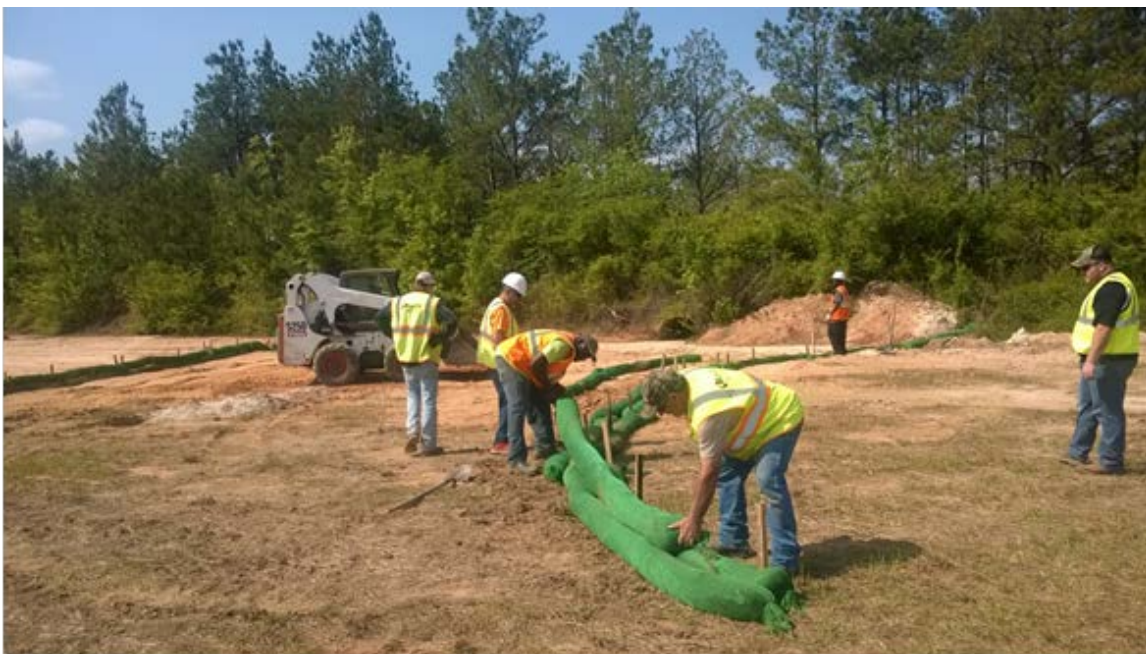
Figure 1. Reactive filter barrier technology being used at Fort Jackson, SC
