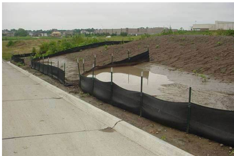
Figure 36. Example of the Use of a Silt Fence as a Best Management Practice for Sediment Control in Runoff Water from a Construction Site.
