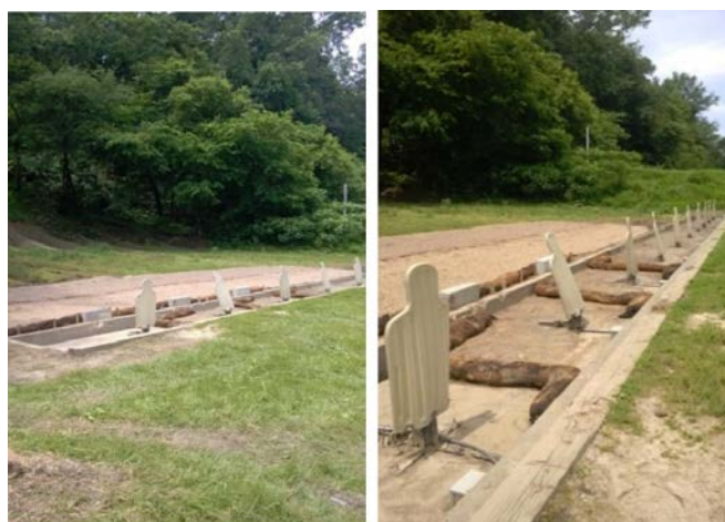
Figure 19. Layout of Reactive Filter Barriers on Center Kinder Range, Fort Leavenworth, KS.
