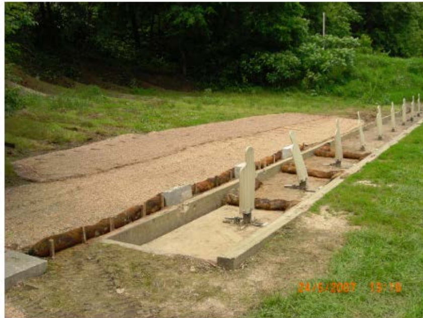
Figure 23. Post-construction Installation of the Reactive Filter Barriers on Center Kinder Range, Fort Leavenworth, KS.
