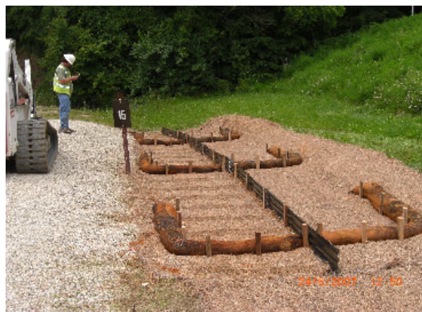
Figure 3. Positioning of the Reactive Filter Barriers in the Flowpath of Range Runoff Water on North Kinder Range, Fort Leavenworth, KS.
