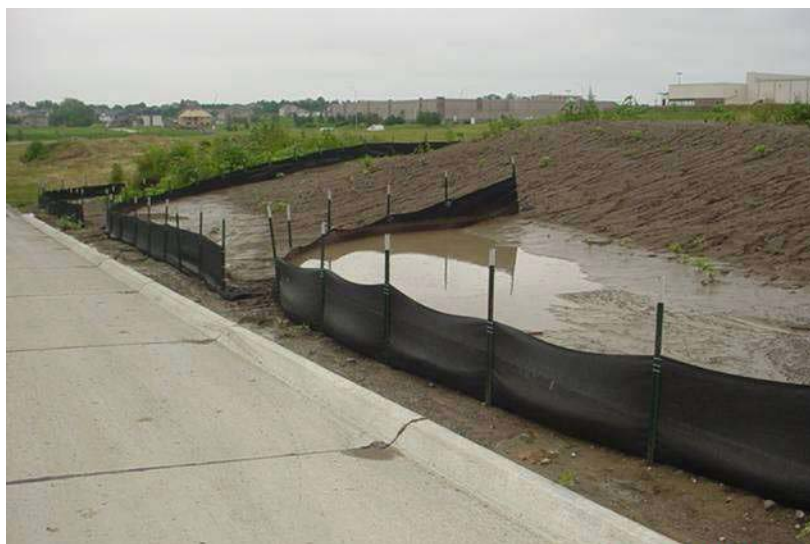
Figure 4. Example of the Use of a Silt Fence as a Best Management Practice for Sediment Control in Runoff Water from a Construction Site.
