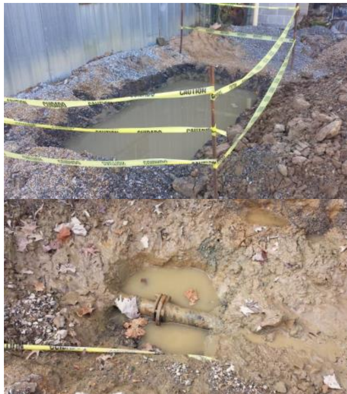
Figure 6-13. Excavation of the Large Leak Identified at ERDC
