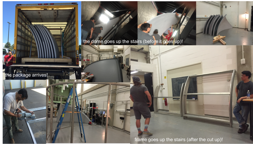
Figure 3: SOLAR system installation process
