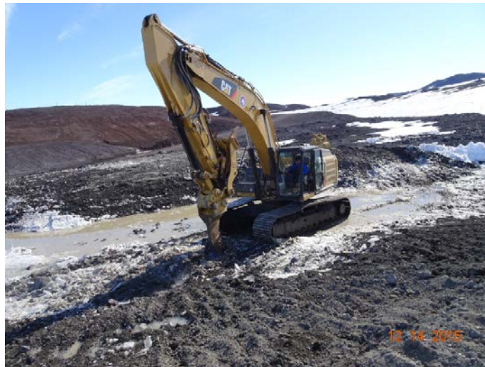
Figure 13. Digging the primary pond at Pond 3C.
