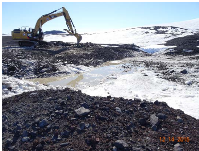
Figure 14. Digging the secondary pond.
