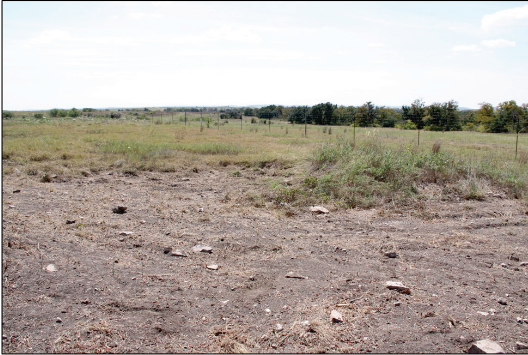
Figure 17. Excessive disturbance with mulching head used for clearing. This level of disturbance excavated stems and roots prohibiting reassessment within the vegetation treatment areas.
