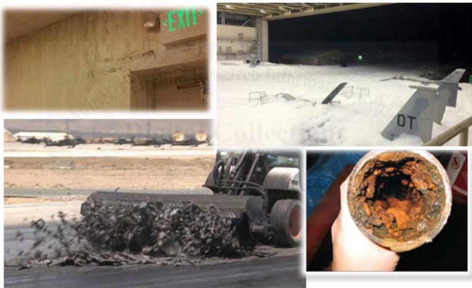
Figure 4: Facility Infrastructure Pictures (Reprinted from AF/A4C Database)
