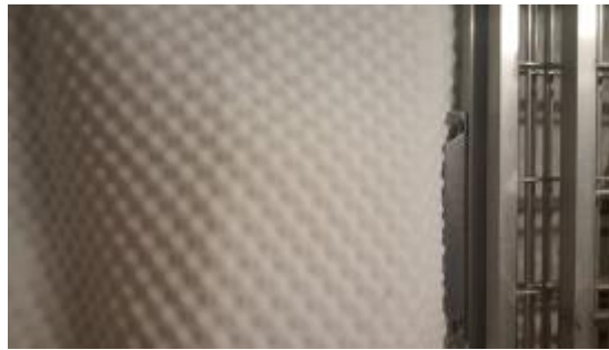
Figure 10: Entrance door to the building covered with polyurethane foam.
