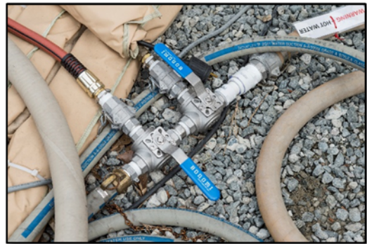
Figure 10: Two Three-way Valves
