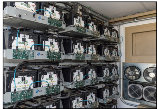
Figure 36: Inverter/Battery System
