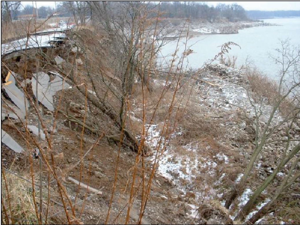
Figure 2. 2004 Bank erosion in problem area.
