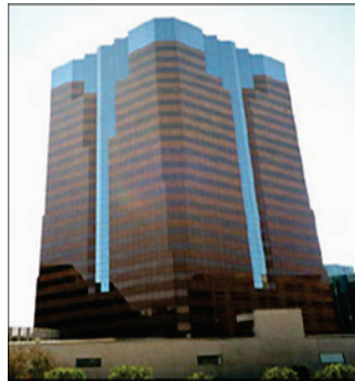
Figure 30. Example of steel moment frame building.
