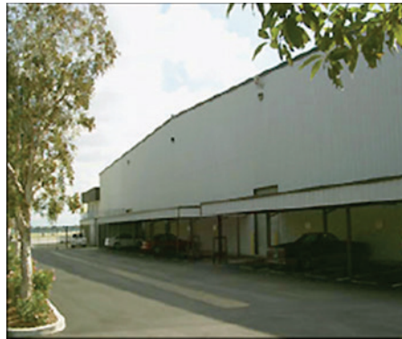
Figure 35. Example of pre-engineered metal frame building.
