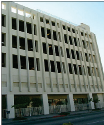
Figure 33. Example of concrete moment frame building.
