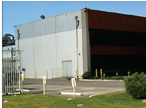
Figure 39. Example of precast/tilt-up concrete walls building.
