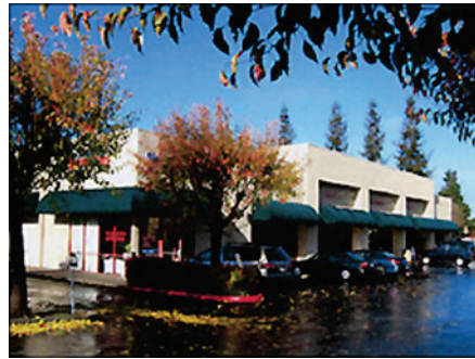
Figure 42. Example of cast-in-place concrete walls building.
