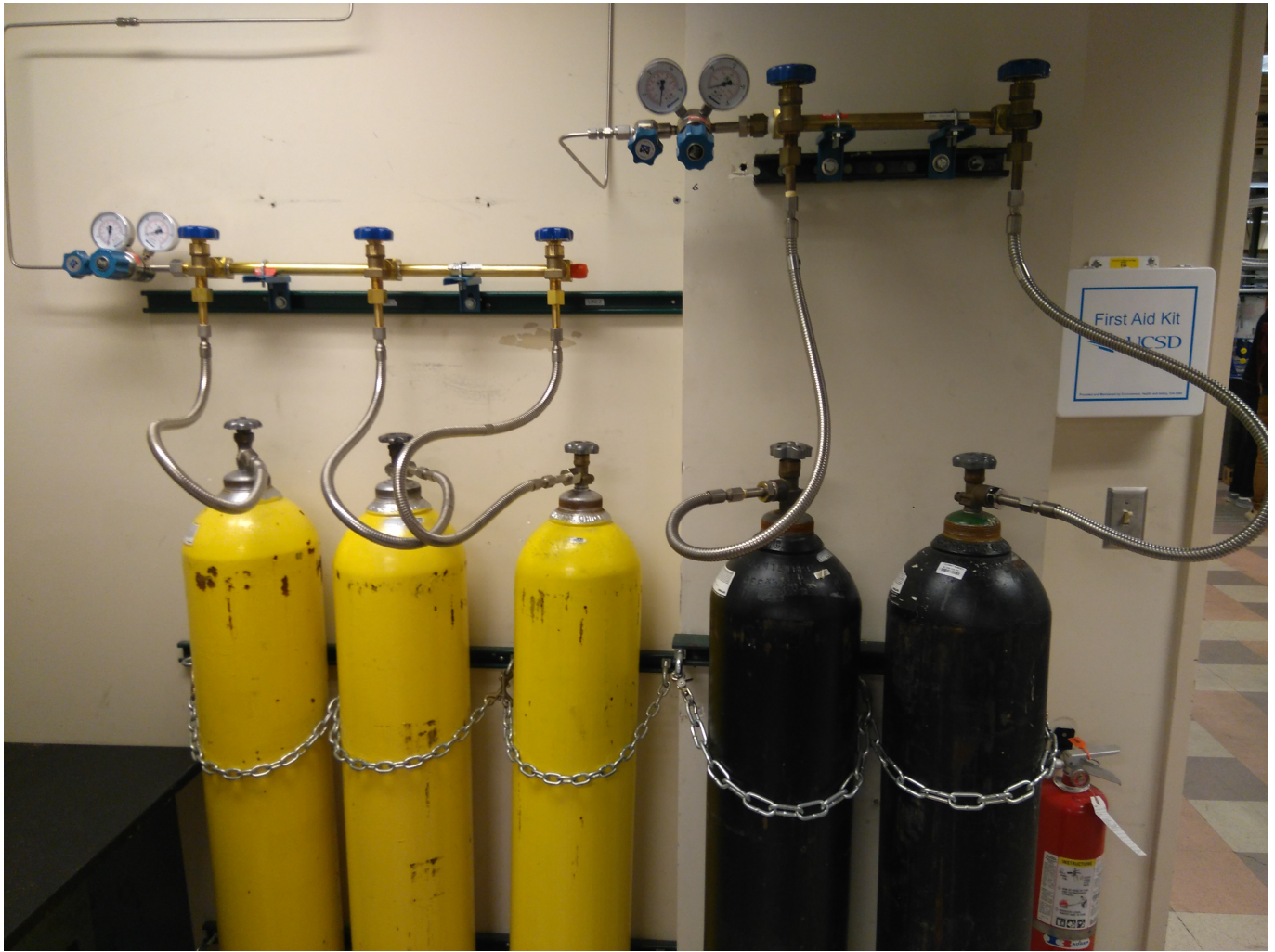
Figure 5: Photo showing two nitrogen gas cylinders attached to a double manifold and three air cylinders attached to a triple manifold.
