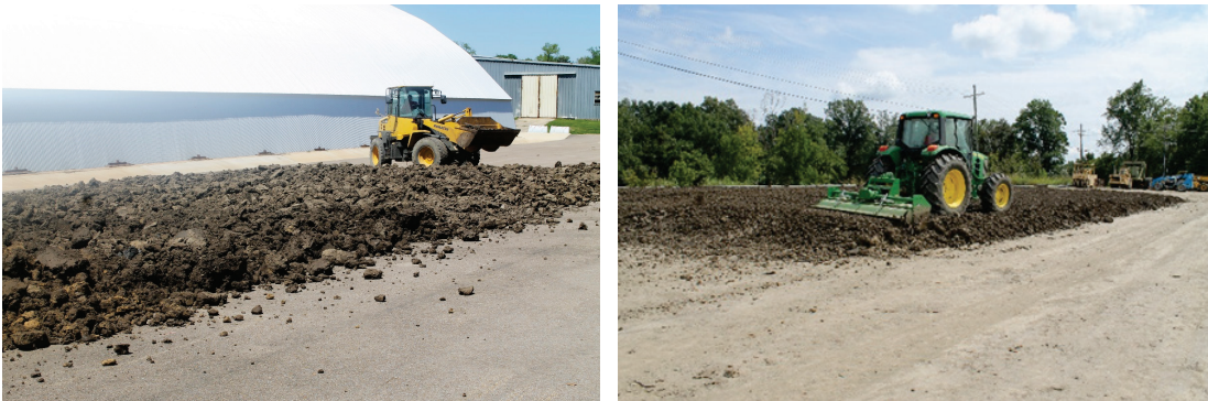
Figure 3.3. Laying out and pulverizing CH to improve moisture consistency.
