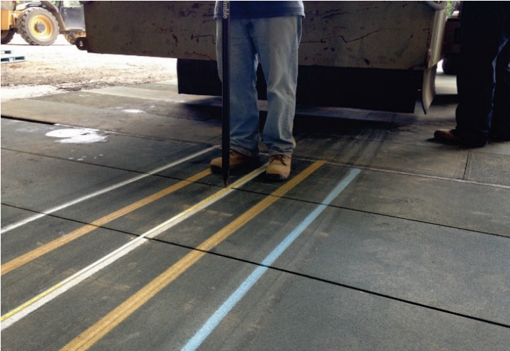
Figure 3.19. Surveying centerline profile.
