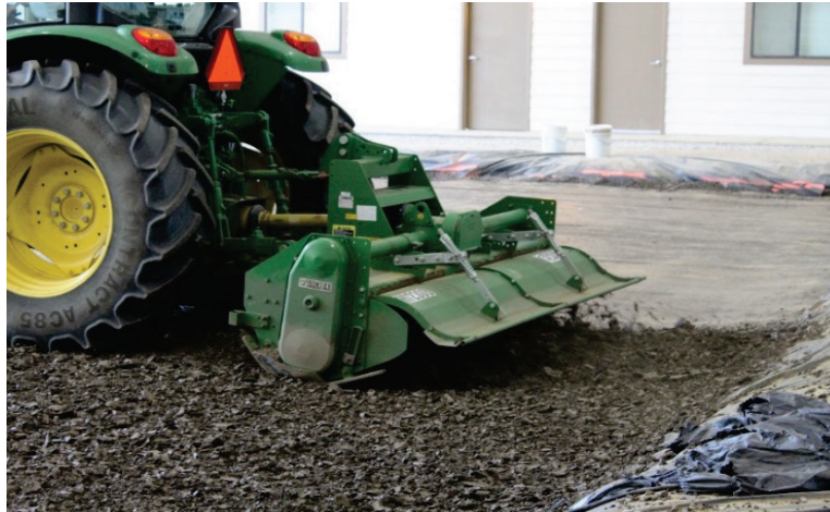
Figure 3.6. Scarifying a lift after installation.
