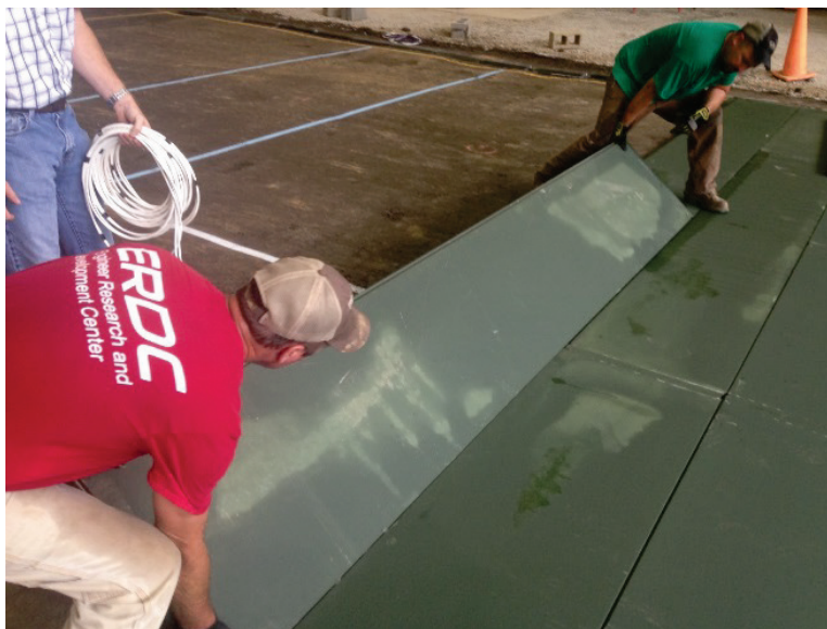
Figure 3.10. Hinging AM2 panel into place.
