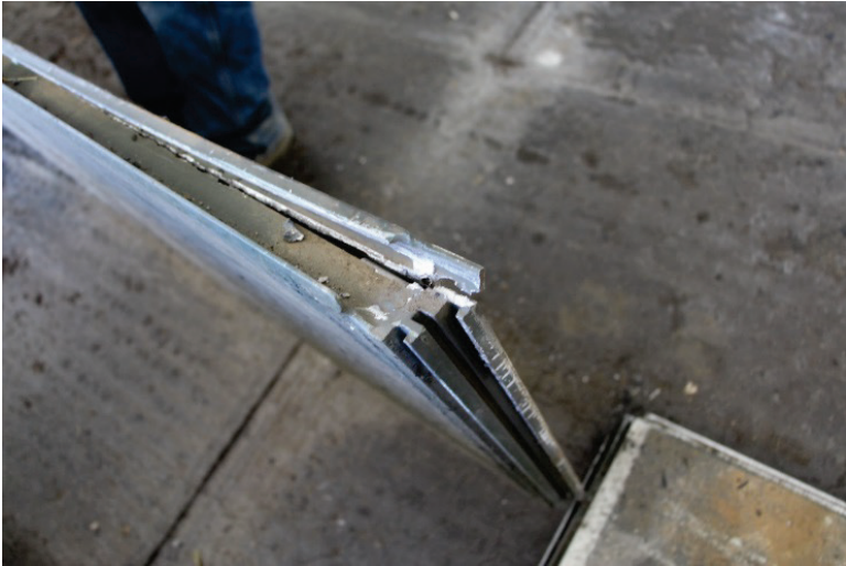
Figure 5.1. 17 in. female hinge crack on panel 2.
