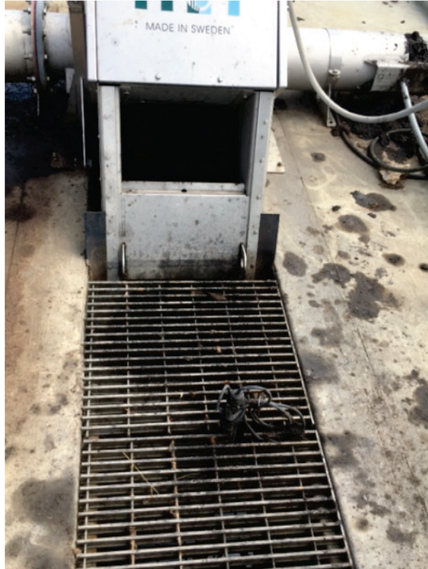
Figure 2. Discharge point from the TanTec facility showing the screen for removal of large constituents.
