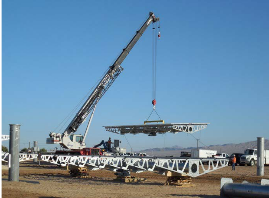
Figure 34. Tracker Table Lift and Installation on the Mast
