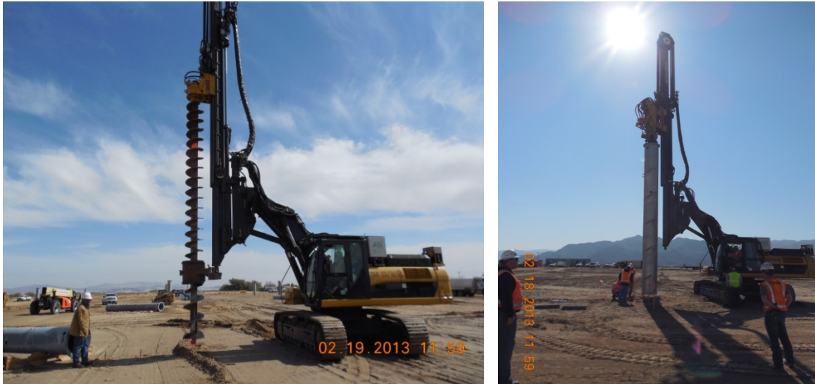
Figure 37. Pre-drilling and driving CPV masts
