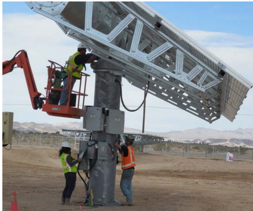
Figure 35. Completion and Commissioning of the CPV System
