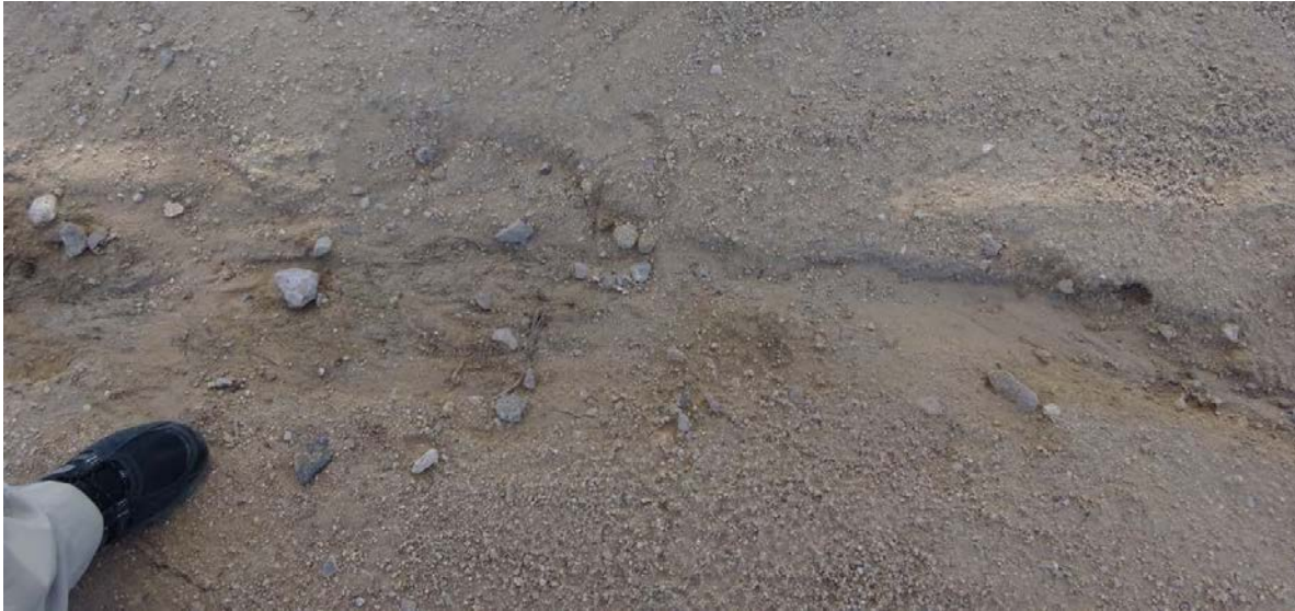
Figure 3 Erosion in the aggregate due to a recent storm. The shoe shown in the picture provides a relative scale for judging the erosion. Plant maintenance personnel indicated that recent storms were strong for the region.
