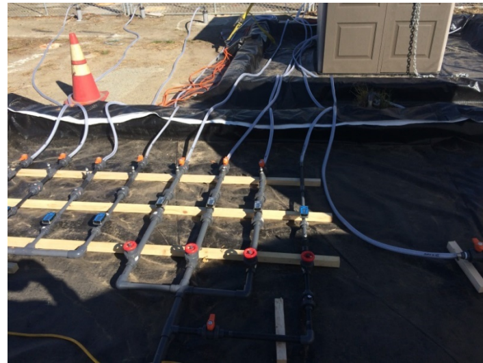
Figure 5.2 Groundwater Recirculation and Tracer Delivery System
