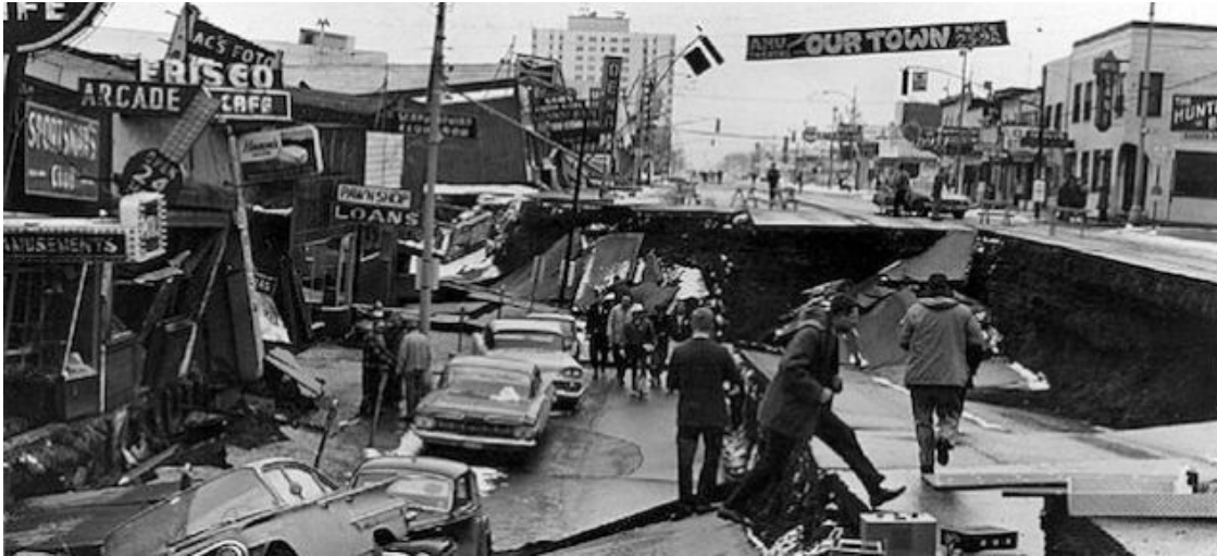
Figure 2 Image source: United States Geological Survey website. Photo of Anchorage after the 1964 earthquake (Survey, 1995). Additional pictures from the USGS of the devastation can be found in Annex A.
