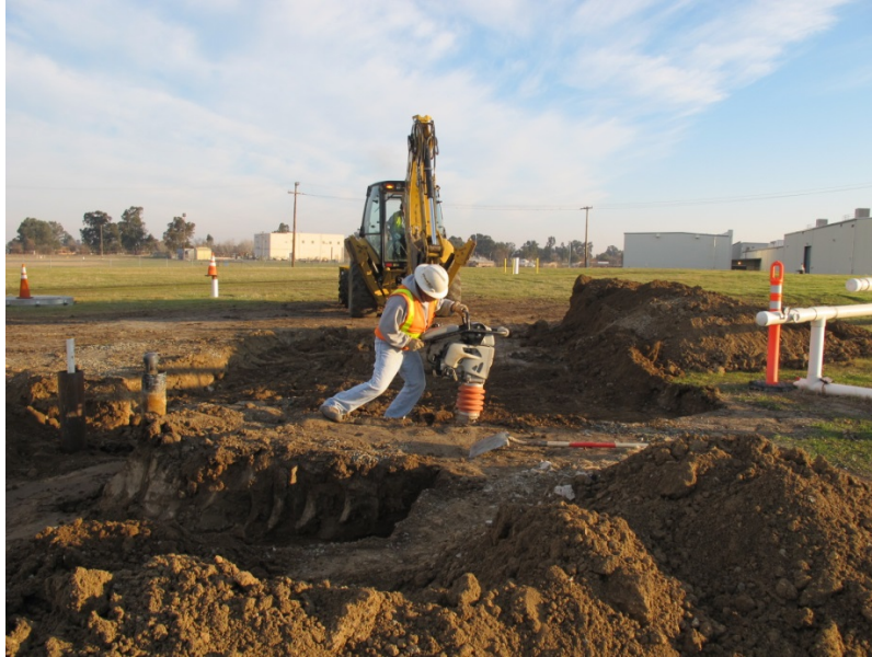
Photo 7. Backfill and compaction.
