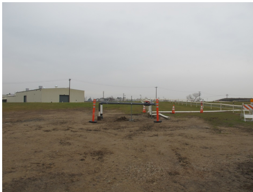
Photo 8. Site after cap restoration.
