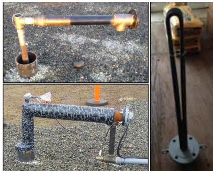
Figure 5.4.4. Injection Wellheads
