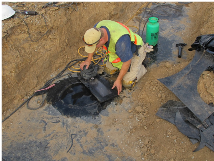
Photo 4. Vacuum Test on a patch.
