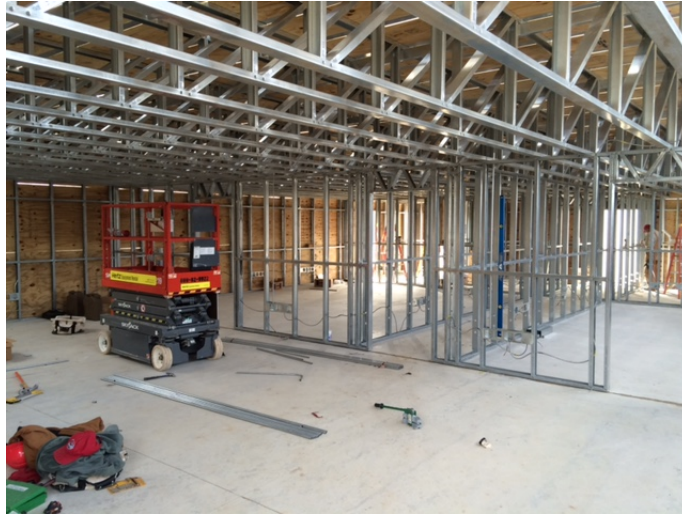
Figure 2.16: FrameCAD Facility Interior - Ft. Bragg, NC [5]
