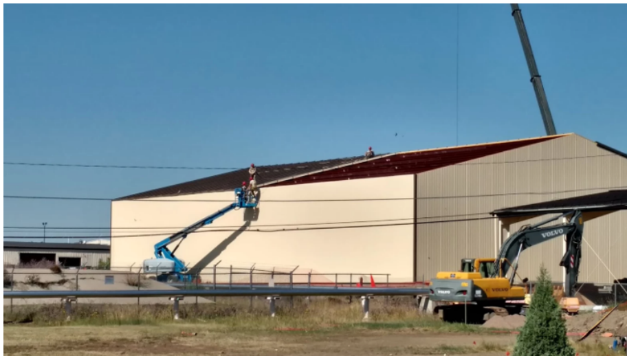
Figure 2.19: PEB Under Construction by 819 RHS - Malmstrom AFB, MT
