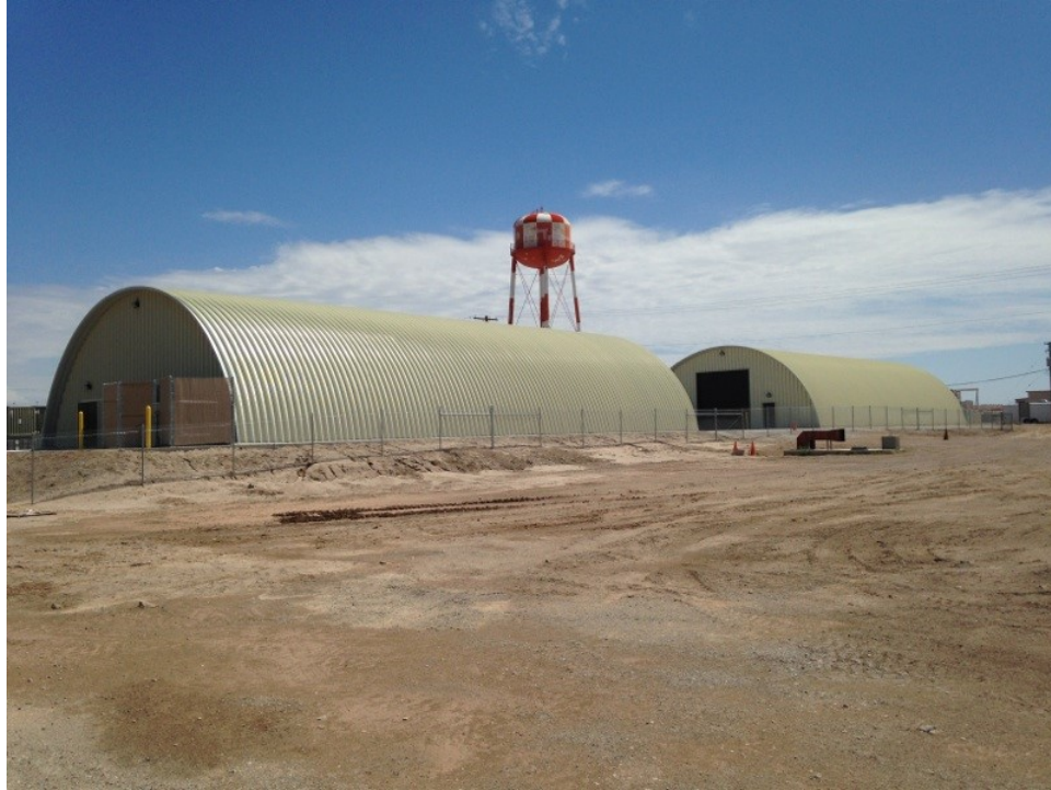
Figure 2.12: Yuma Proving Grounds K-Spans - YPG, AZ [4]
