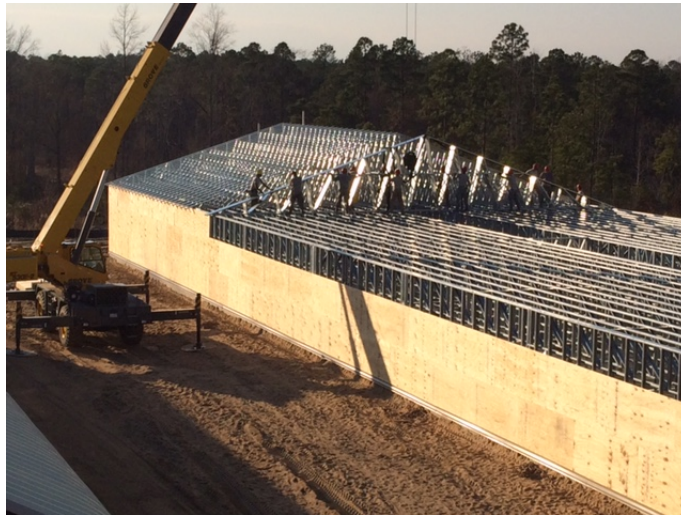
Figure 2.15: FrameCAD Facility Sheeting Process - Ft. Bragg, NC [5]
