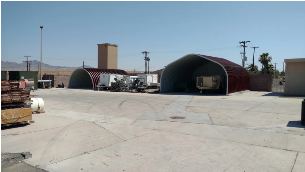
Figure 2.6: Type 1 and 3 K-Spans - Nellis AFB, NV
