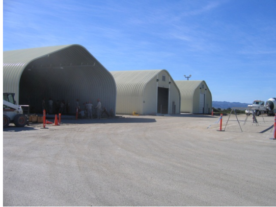
Figure 2.5: Type 3 K-Spans - Vandenberg AFB, CA [1]
