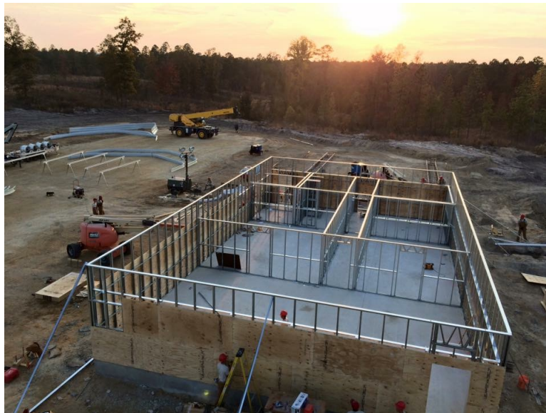
Figure 2.17: FrameCAD Facility Top View - Ft. Bragg, NC [5]
