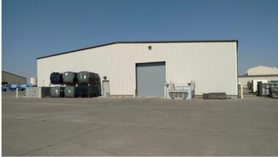
Figure 2.20: PEB Facility - Malmstrom AFB, MT
