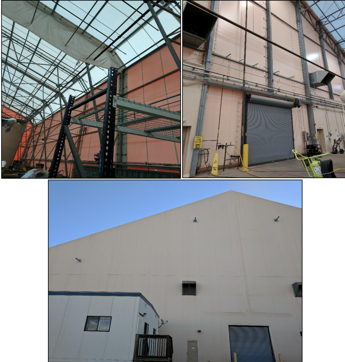
Figure 4 Photos taken at Hangar A
