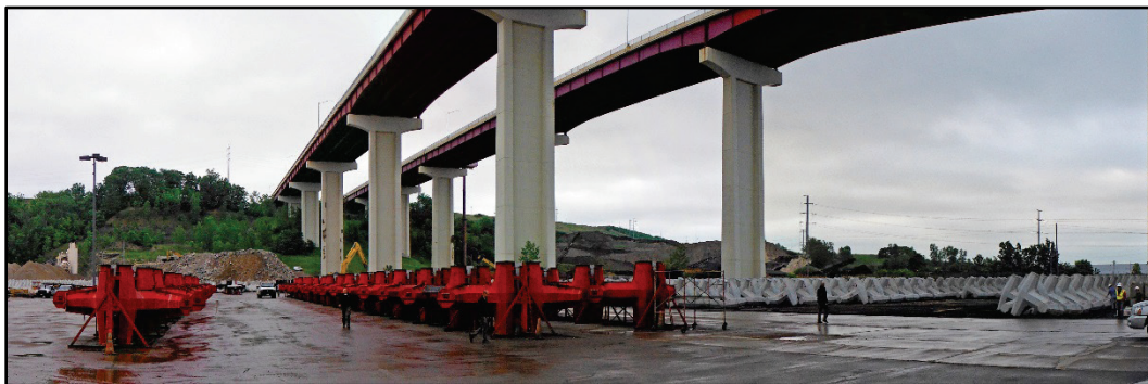
Figure 3-15. Ground view of Allegra Concrete forms and curing dolosse, June 2015.
