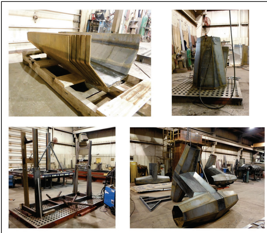
Figure 3-1. Constructing Cleveland 6.5-ton dolos forms.
