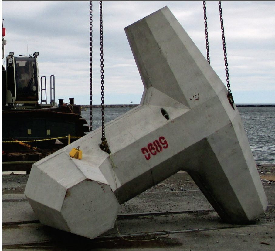
Figure 3-12. Lift method when moving Oswego 16-ton dolos.
