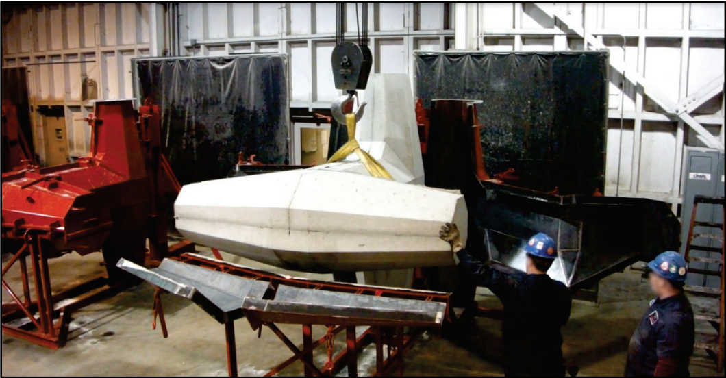
Figure 3-10. Lifting Cleveland 6.5-ton dolos out of form.
