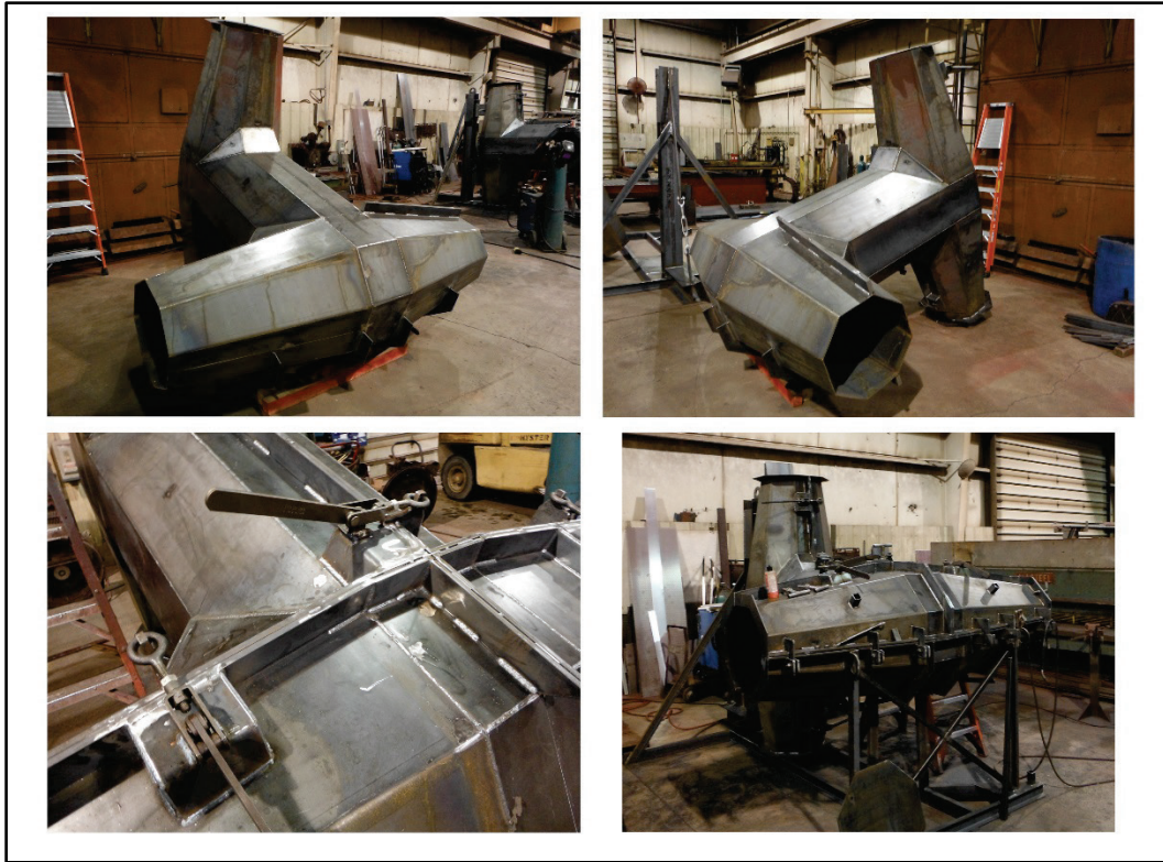
Figure 3-2. Constructing Cleveland 6.5-ton dolos forms.
