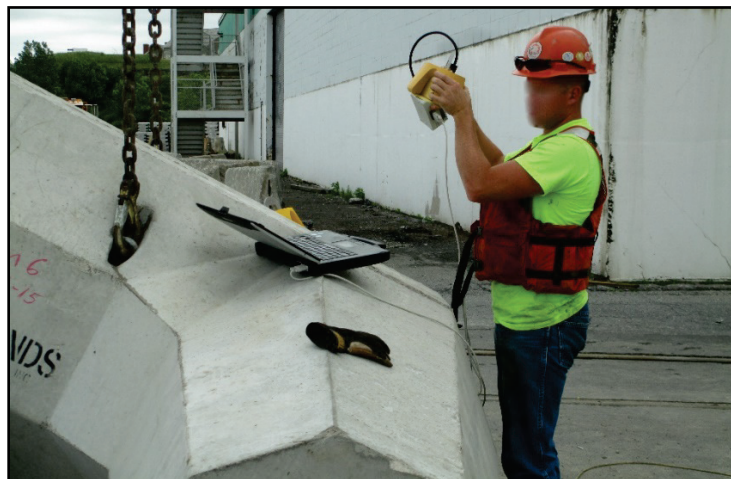
Figure 4-7. Calibrating BIB on Oswego dolos.
