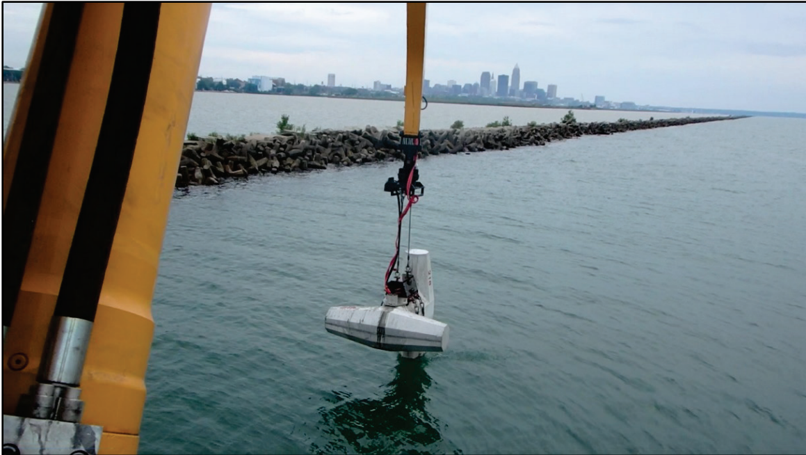
Figure 4-11. Placing saddle from Cleveland dolos at toe of section (video time 1:32 min:sec).
