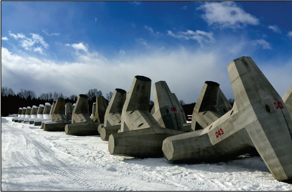
Figure 3-16. Lakeland storage yard for Oswego 16-ton dolosse, February 2015.
