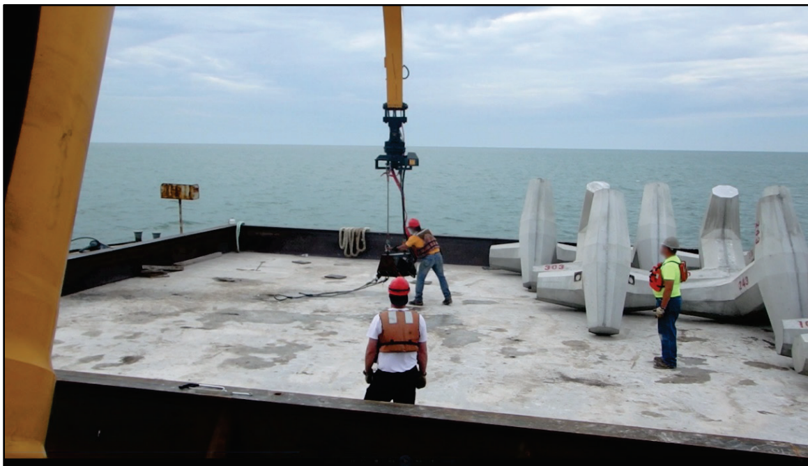
Figure 4-12. Cleveland dolos lifting mechanism returns for next dolos (video time 4:17 min:sec).
