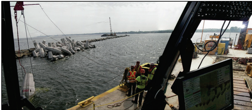
Figure 4-2. Crane operator's view of Oswego dolos placement.
