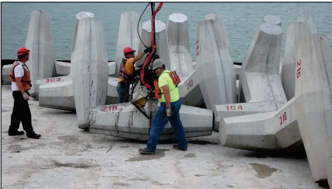
Figure 4-10. Removing saddle from Cleveland dolos prior to lifting (video time 0:21 min:sec).
