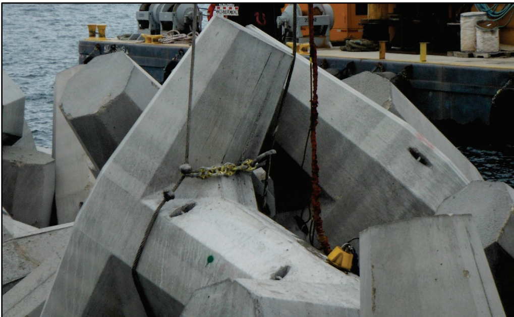
Figure 4-15. Oswego dolos lifting arrangement.
