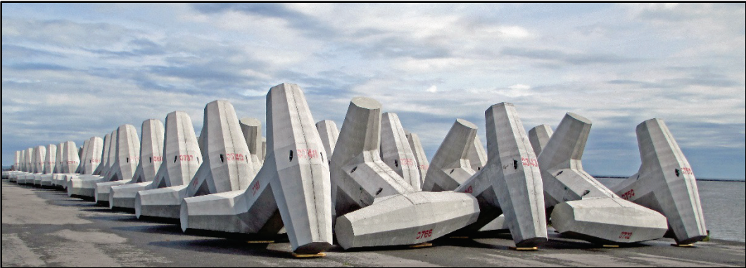
Figure 3-24. Dolosse at Port of Oswego, New York.
