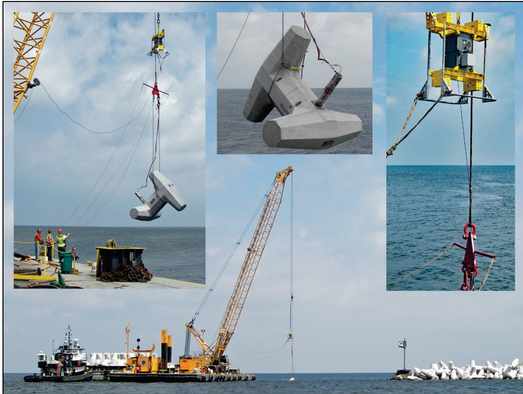
Figure 4-16. Oswego dolos lifting arrangement.
