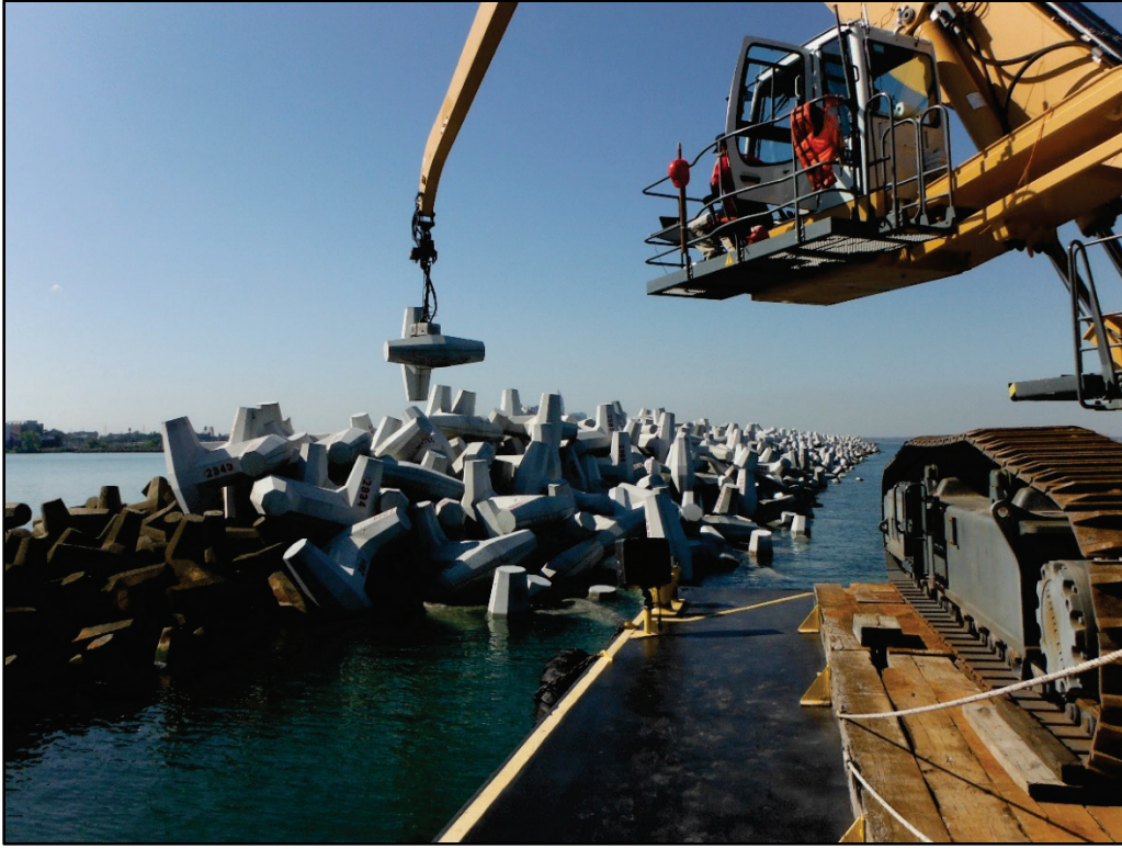
Figure 4-14. Placing Cleveland dolos.
