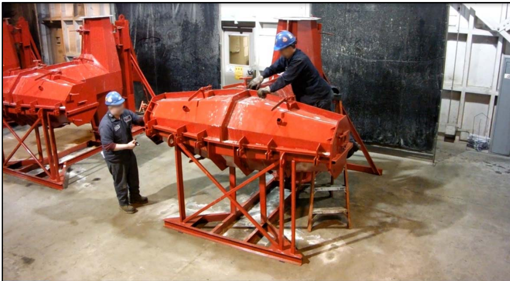
Figure 3-7. Loosening bolts and opening latches on Cleveland 6.5-ton dolos form.
