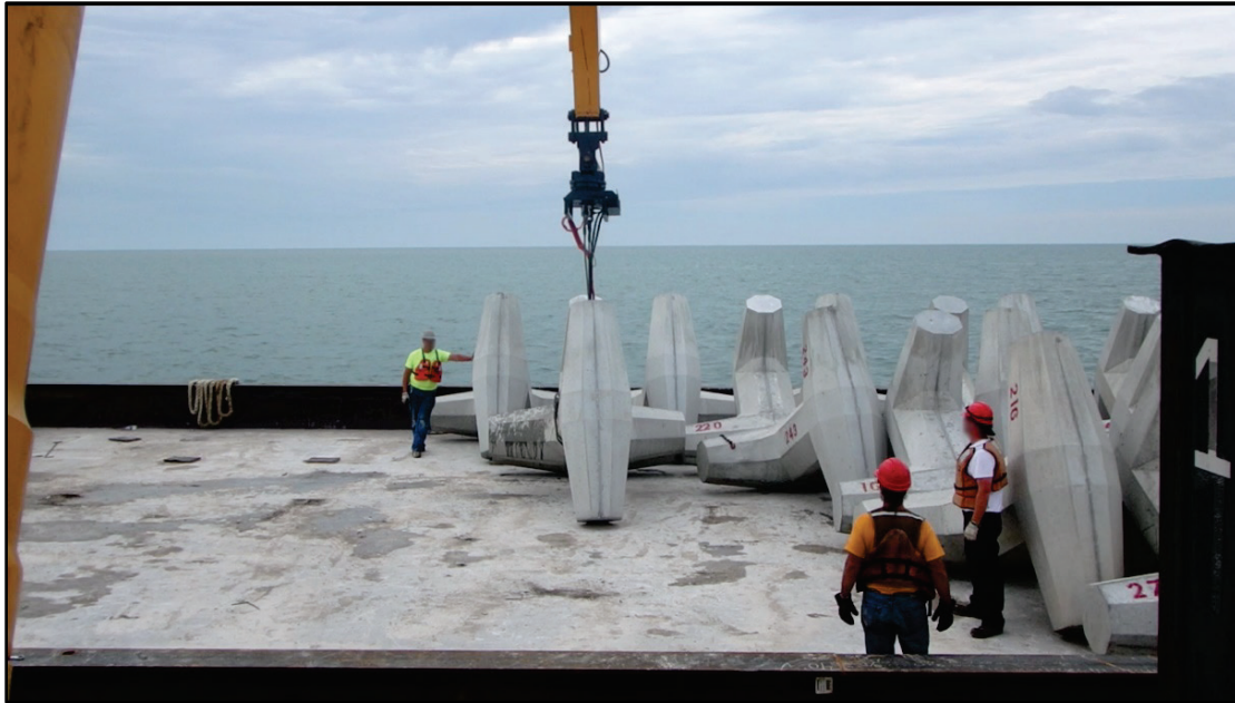
Figure 4-13. Next Cleveland dolos is being lifted for placement (video time 5:39 min:sec).
