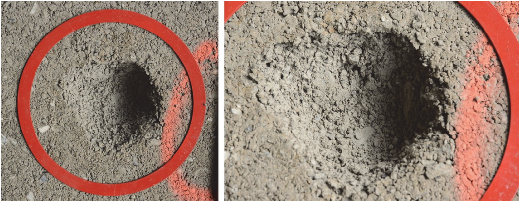
Figure 36. GW-GC-Gravel with silty clay and sand soil excavation.
