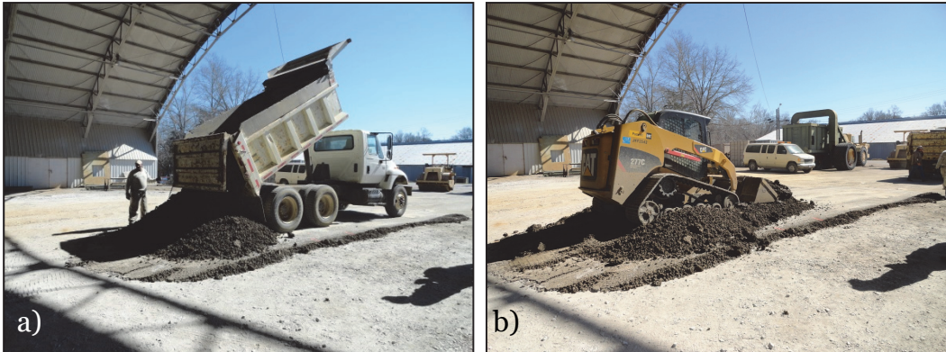
Figure 26. Placing soil to build a testbed using a) dump truck and b) skid steer.
