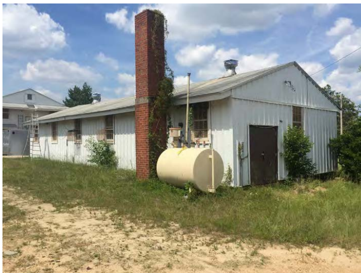
Figure 7. Building A5436 at Fort Bragg Army Base
