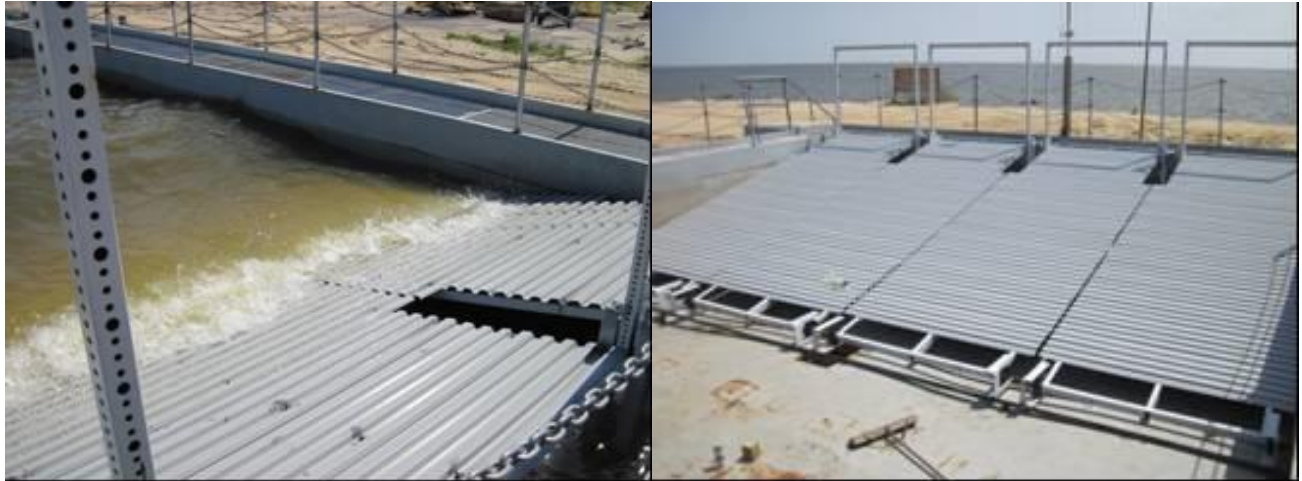
Figure 9. View of energy dissipation beach with (left) and without water (right).
