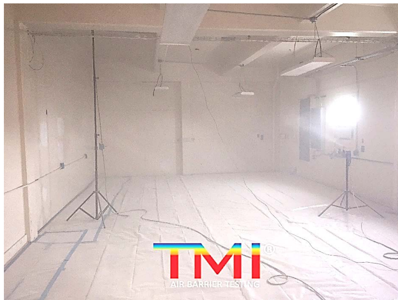
Figure 5. Building 2177 at Quantico Prepped for Aerosol Envelope Sealing
