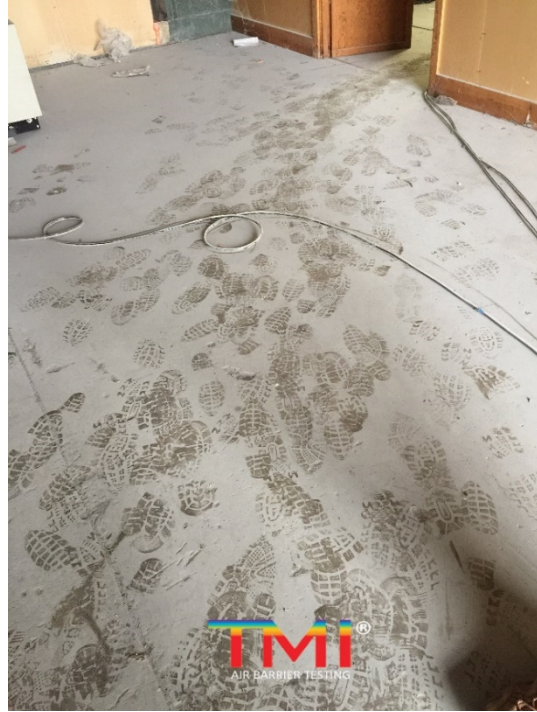
Figure 11. Photo Showing Floor Prepped at Ashurst Elementary at MCB Quantico (left), and Floor Not Prepped at Building 608A at NSA Mechanicsburg (right)
