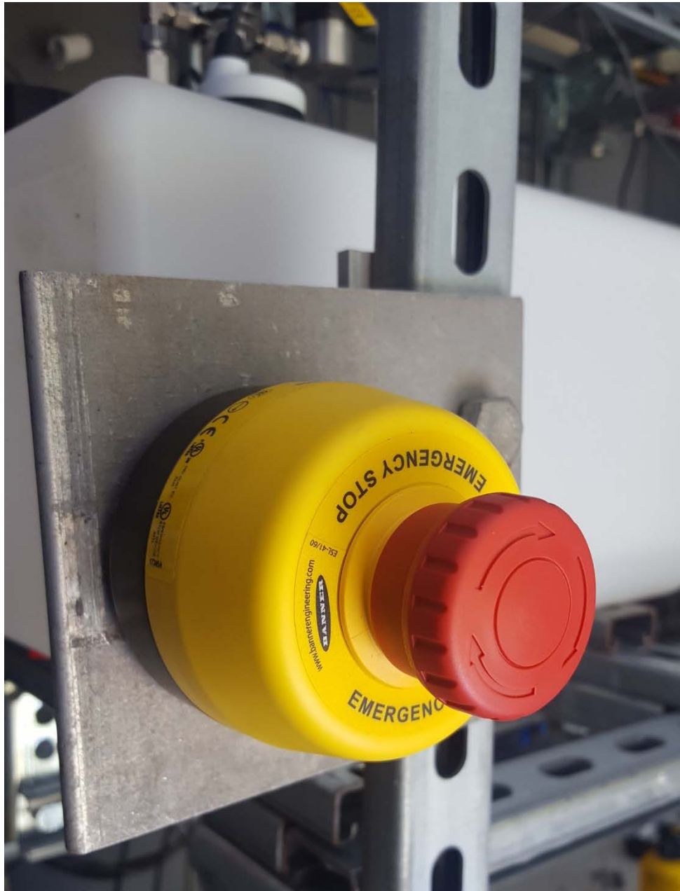
Figure 10. Emergency stop pushbutton.
