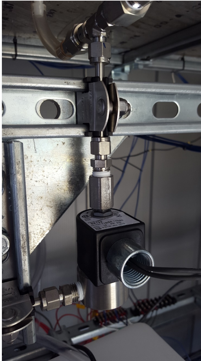
Figure 15. Omega SV133 normally open fluid control valve.
