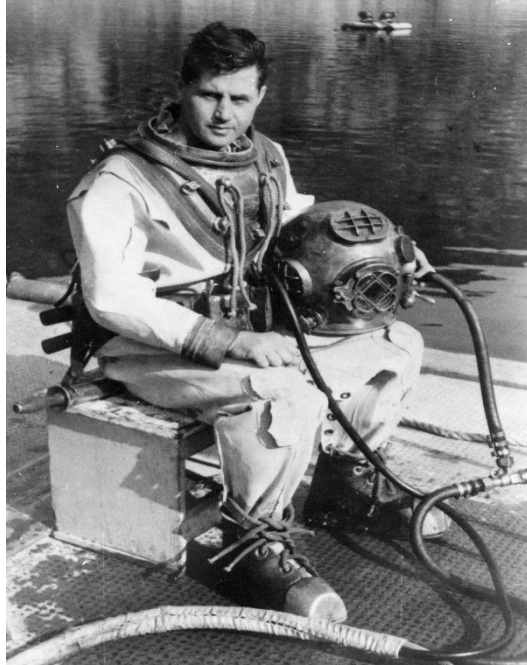
Figure 3. U.S. Navy diver wearing Mark V rig (developed in 1916). Source: [7].
