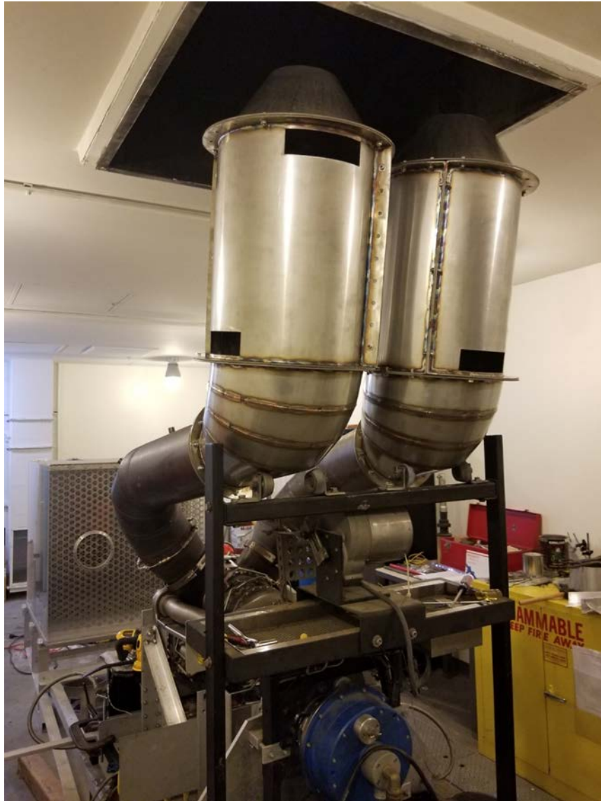
Figure 10. Installed Heat Exchanger Duct
