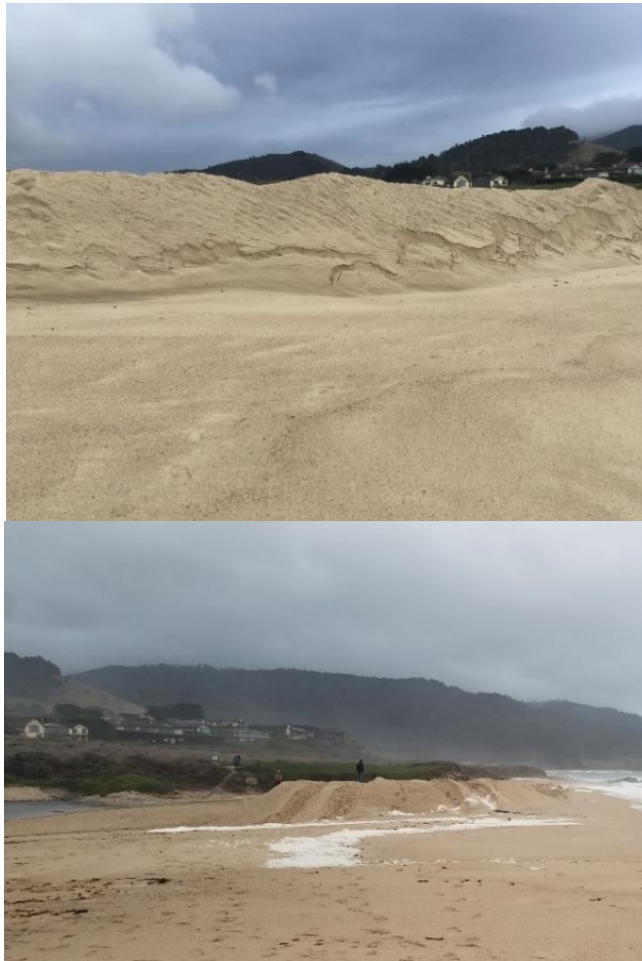
Figure 10. Sand Berm Resulting from Excavation of the Breach.
