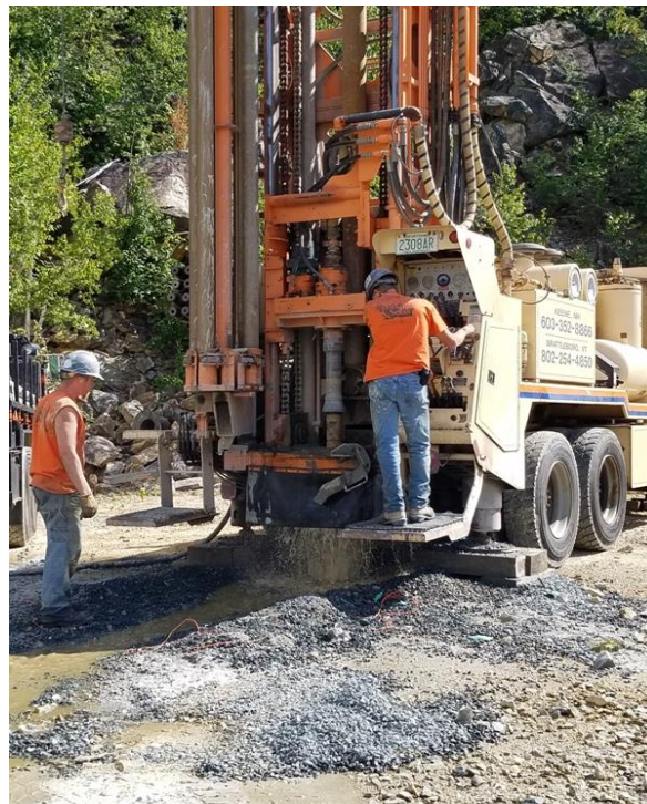
Figure 23. Re-drilling SH7 borehole.
