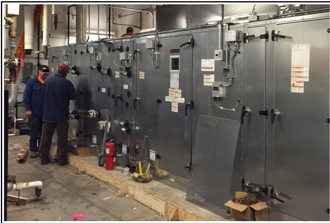
Figure 13. New HEDS AHU in Bldg. A-3556 at Fort Bragg.
