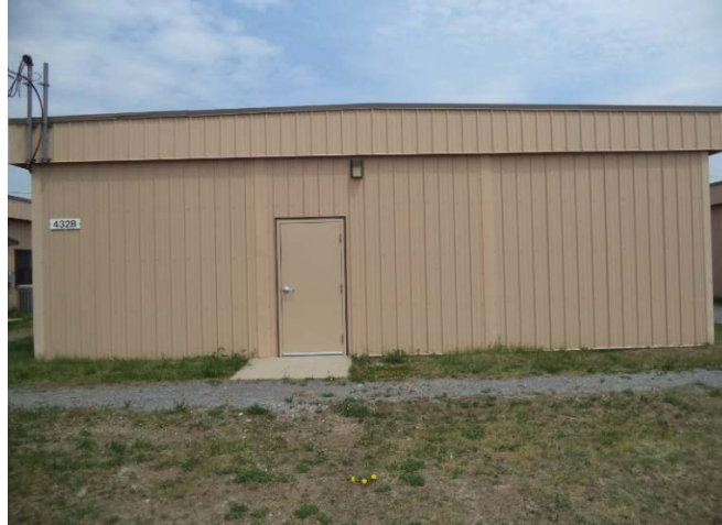
Figure 7. Fort Drum Retrofit Facility.
