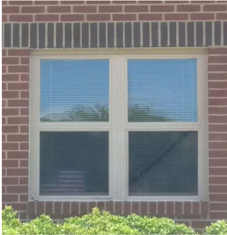
Figure 3-6. Single hung window (4x4-ft) in Bldg 1540A (typical of 10).
