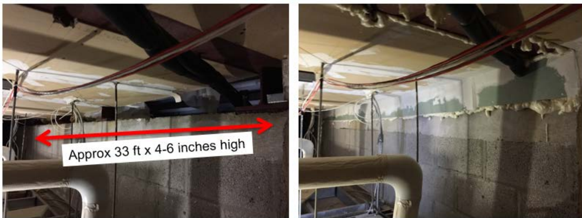
Figure 3-5. Sealing of a major opening above the hard ceiling above the Men's Latrine.
