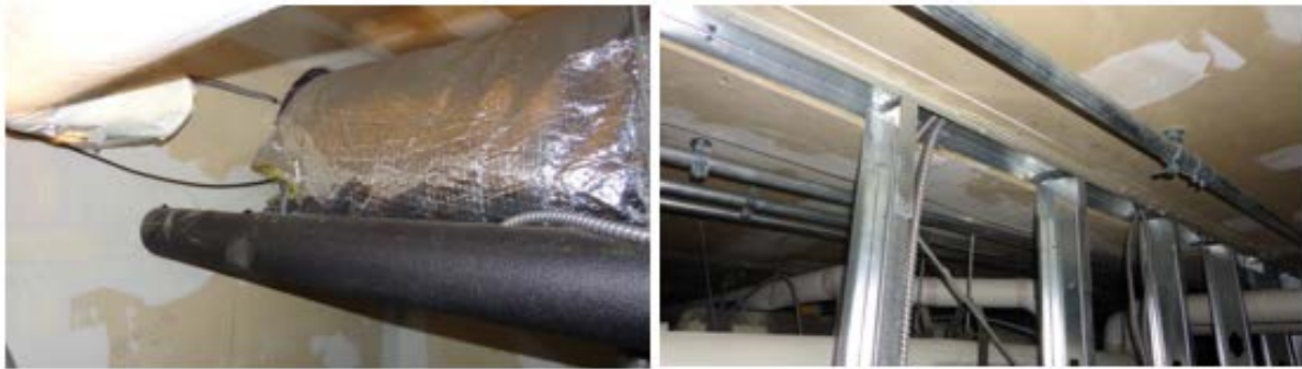
Figure 3-1. Leakage sources at pipe penetrations and at framing systems.
