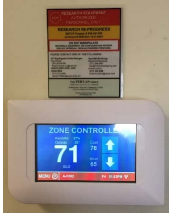
Figure 5-2. Typical EnTouch EMS zone thermostat and temperature/humidity logger.
