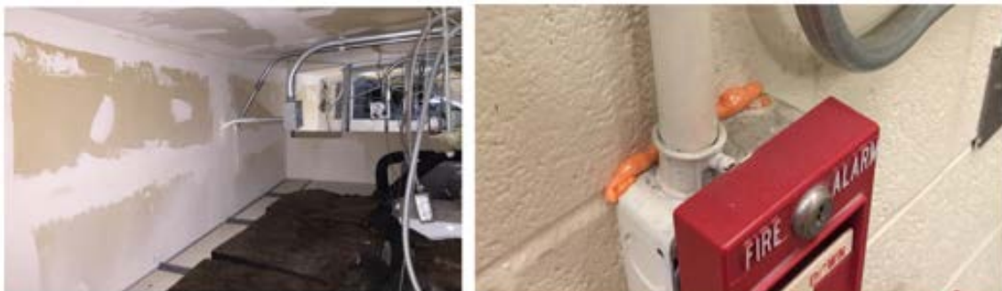
Figure 3-3. Sealing of conduit penetrations in cavity space above the suspended ceiling of Bldg 1540A (left) and at the mounting location of a 4x4 conduit box (right).
