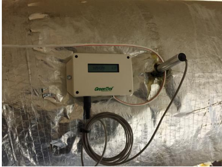
Figure 5-21. Air flow sensor located in AHU-4 supply air.
