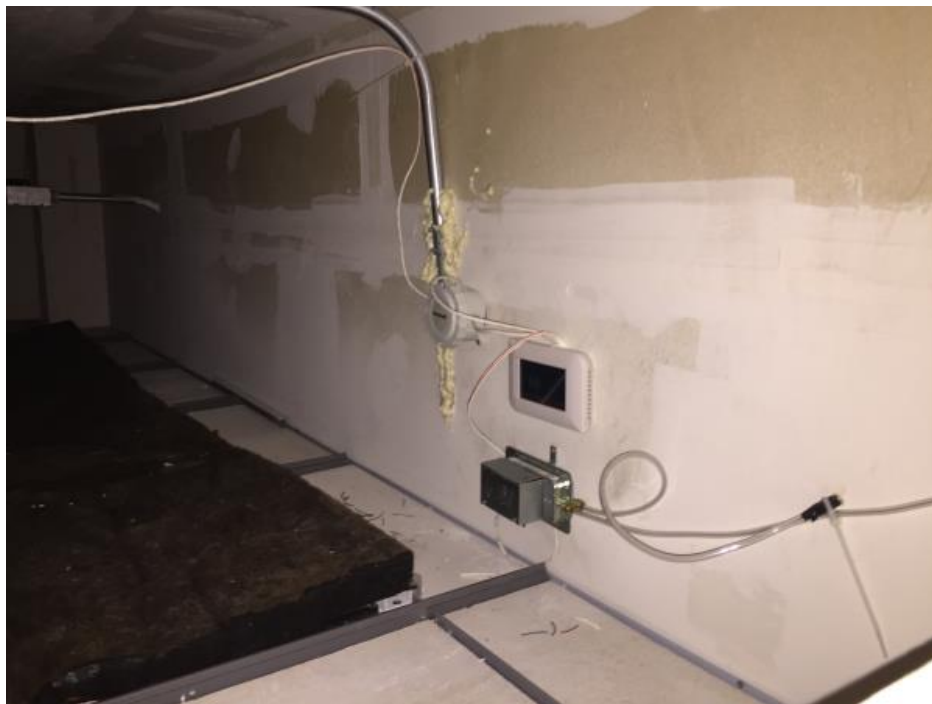
Figure 5-16. Building envelope DP sensor and wall temperature/RH sensors installed above office C003.
