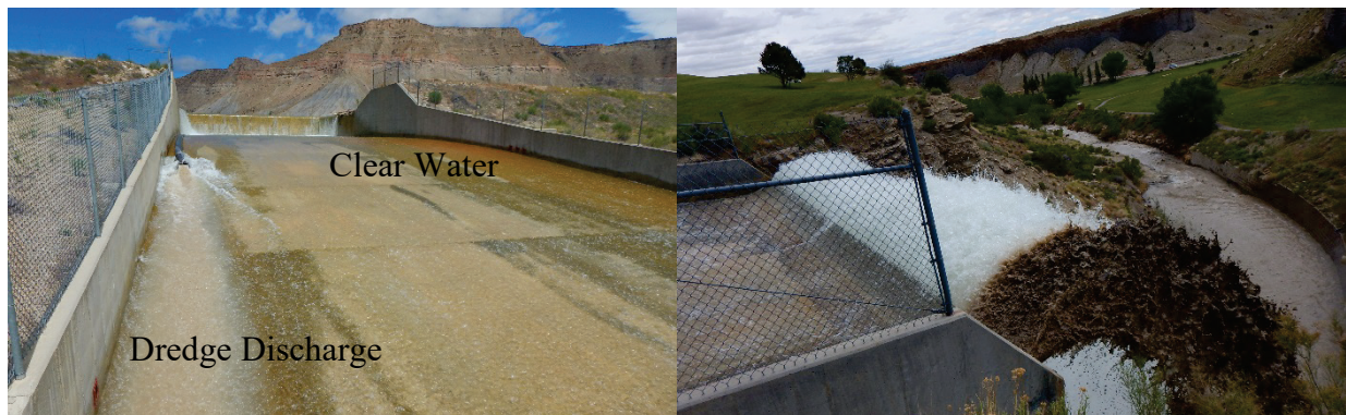
Figure 3. Spillway discharge from Millsite Reservoir (June 2017). The dredge discharge induces the turbid plume.
