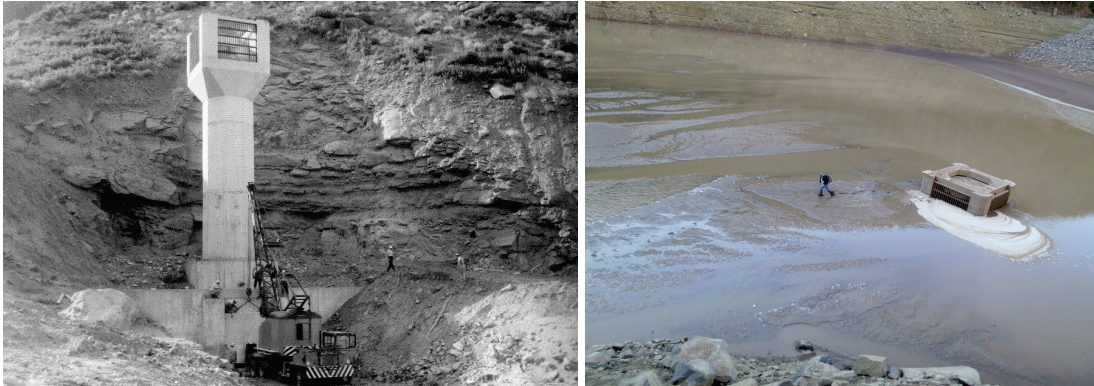
Figure 4. Paonia Reservoir Inlet in 1961 (left) and 2014 (right). Note the individual walking on the sediment in the 2014 picture.
