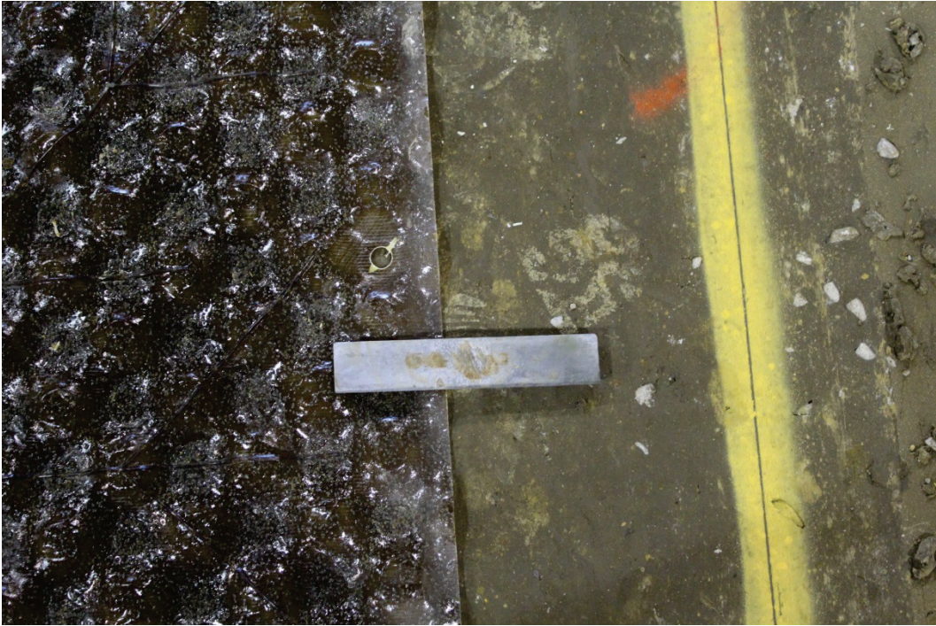
Figure 8. Typical installed T-stake anchor.
