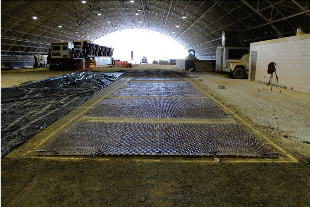
Figure 7. Completed CH-6 test section with WavTrac EMMS.
