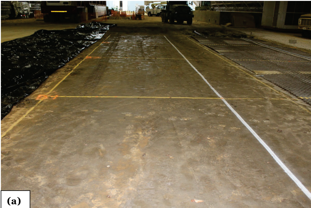
Figure 22. Control test item (a) before and (b) after traffic operations.
