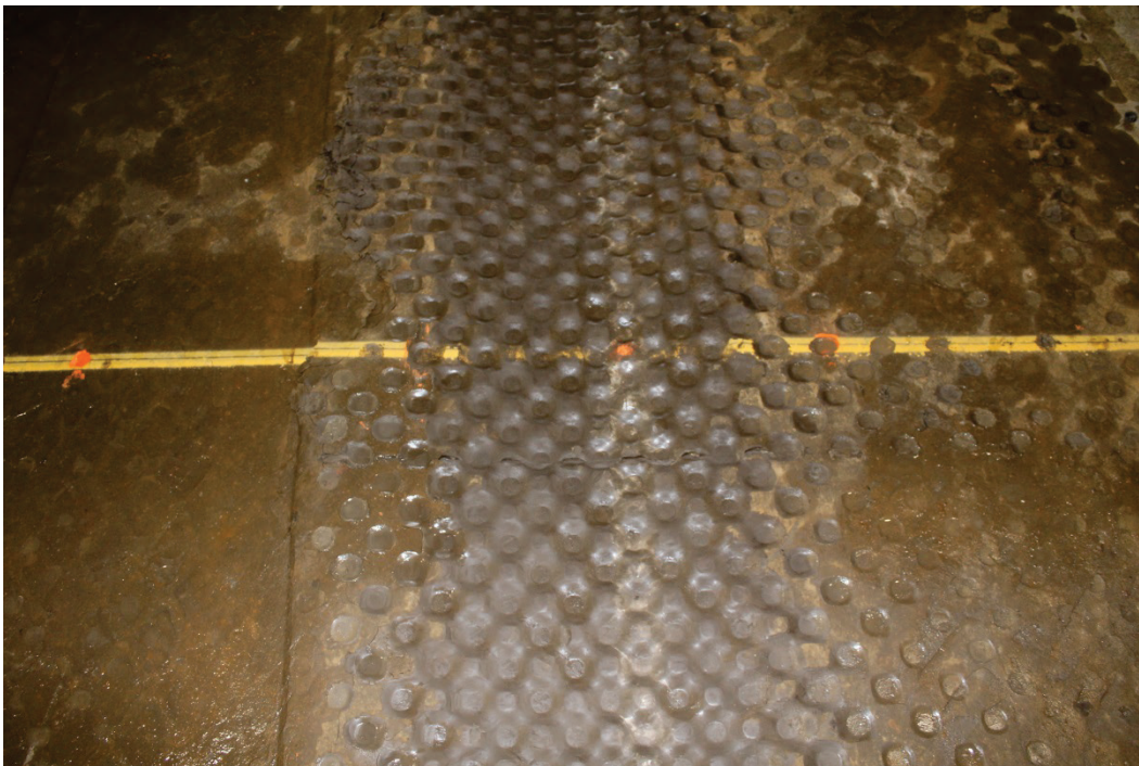
Figure 23. CH-6 subgrade surface following WavTrac removal.
