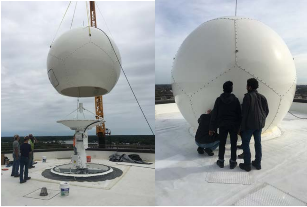
Figure 5.1 Installation of the DBS on HU's Harbor Centre Rooftop.
