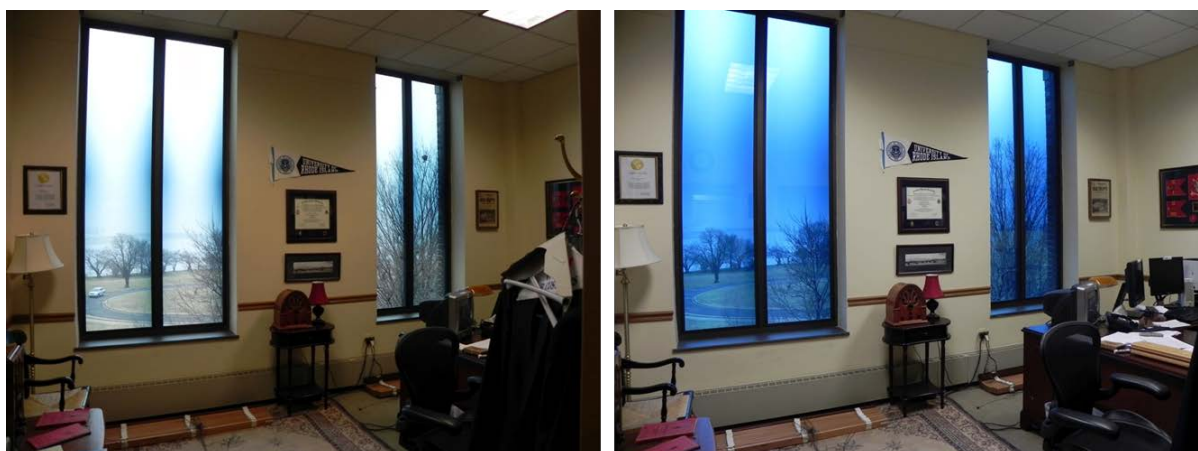
Figure 17. Glass Appearance as Commissioned – during Tint Transitioning
