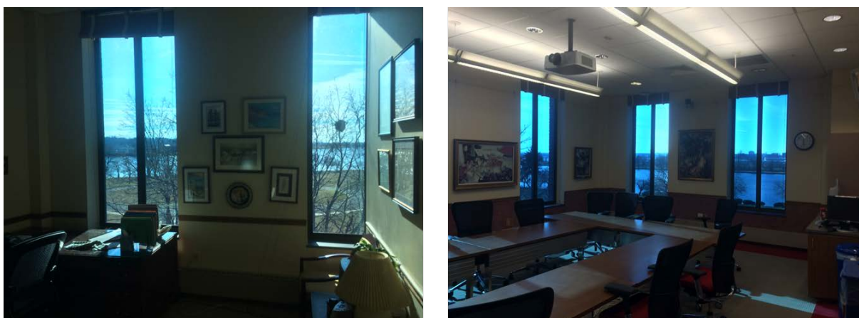
Figure 18. Glass Appearance as Commissioned – Fully Tinted
