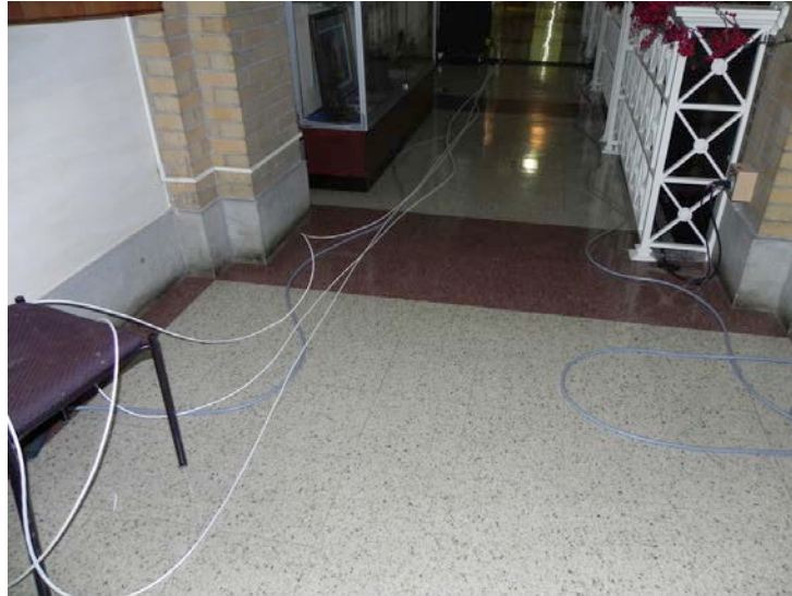
Figure 11. Central Trunk Cables Laid Out in Central Corridors
