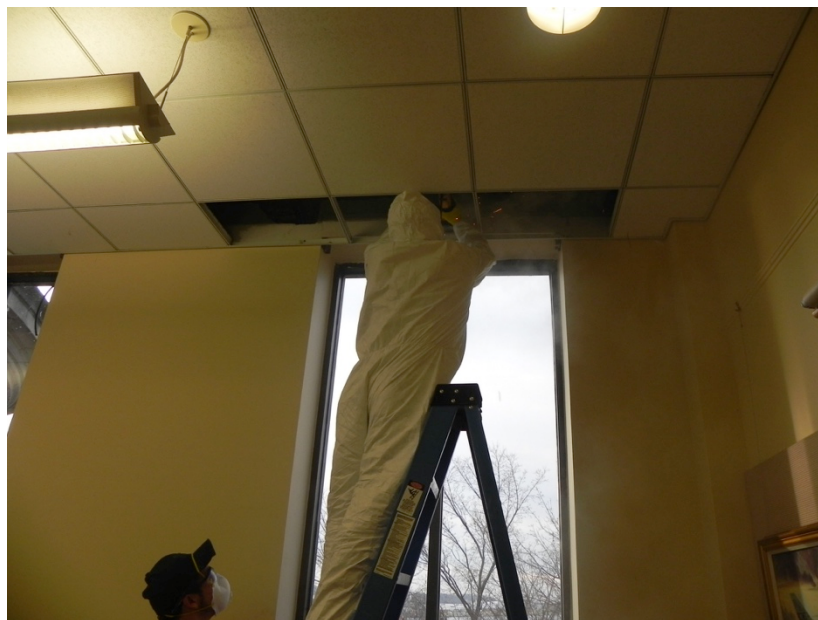
Figure 10. Installation of Dynamic Glass System Components in the Existing Ceiling Plenum
