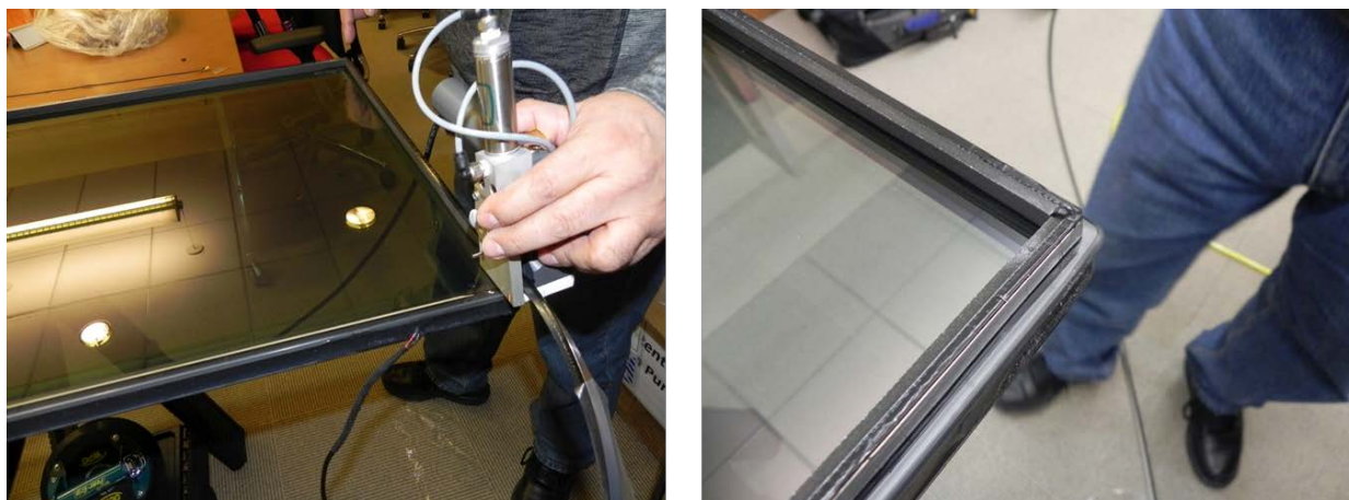
Figure 14. Perimeter Spacer/Seal was Applied at Site
