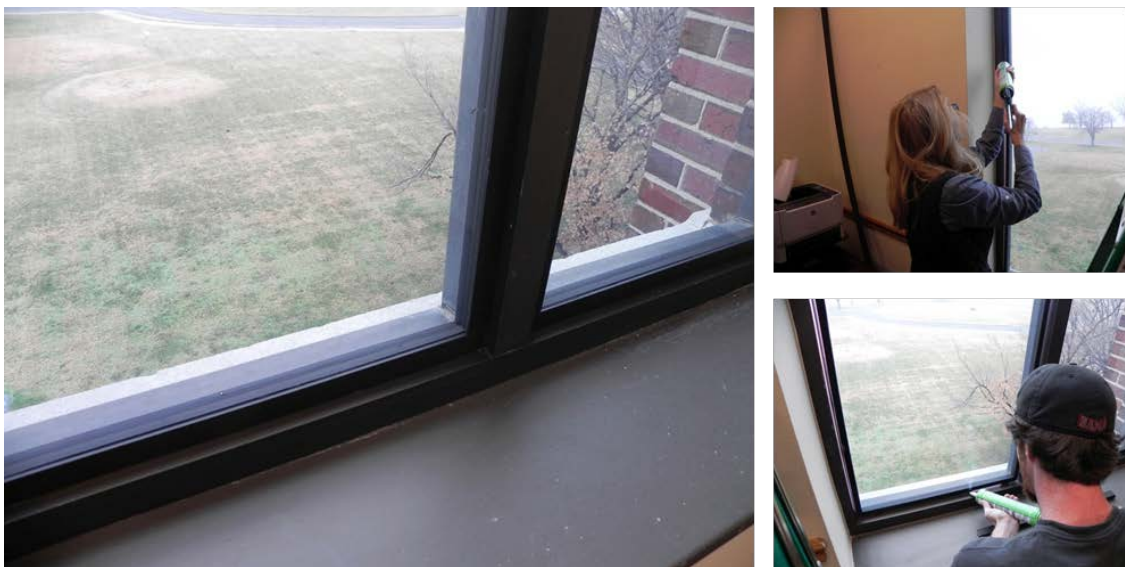
Figure 16. Interior Frame Being Installed and Sealed
