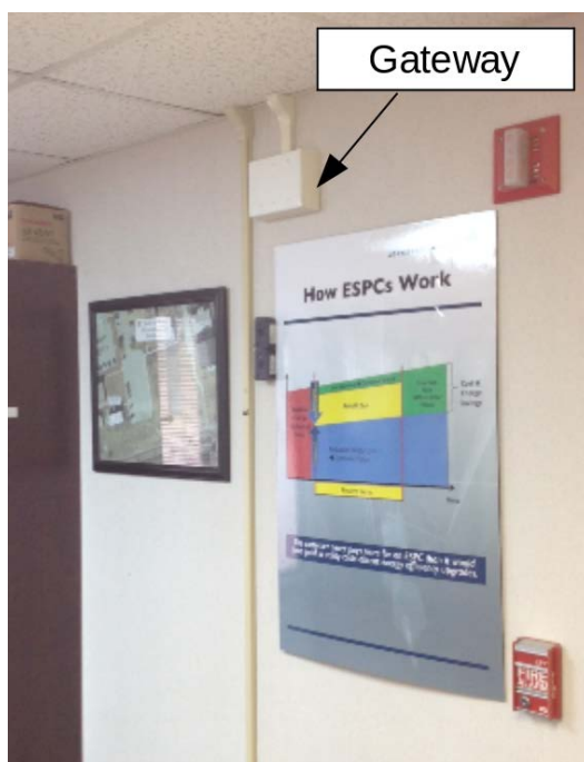
Figure 28. Typical Gateway Mounting
