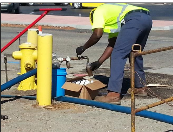
Figure 10. Collecting Samples during Ice Extraction
