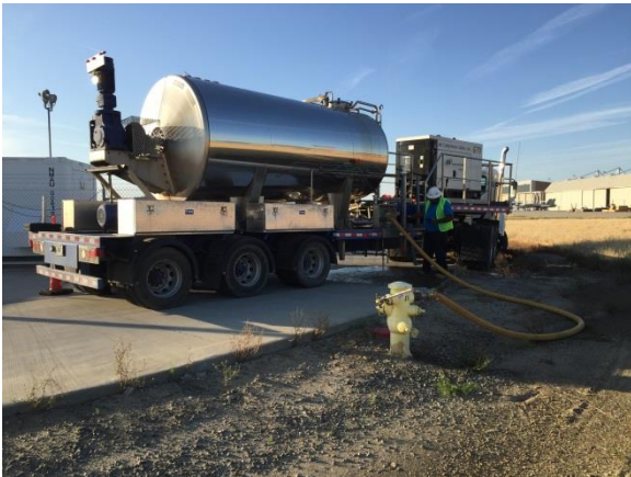
Figure 9. Inserting Ice Slurry into Upstream Hydrant
