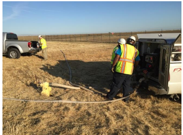
Figure 8. Extracting Ice at Downstream Hydrant
