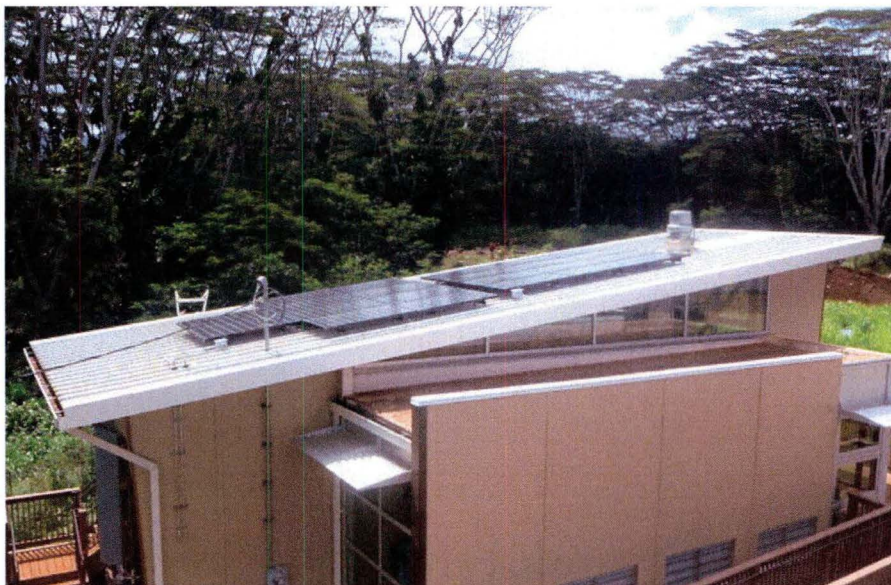
Figure 2. Kawaikini West Building, East Kauai, with heterojunction with intrinsic thin layer (HIT) in a string configuration (top) and monocrystalline with microinverters (bottom).
