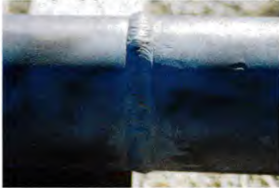
Grit blasted pipe weld.
