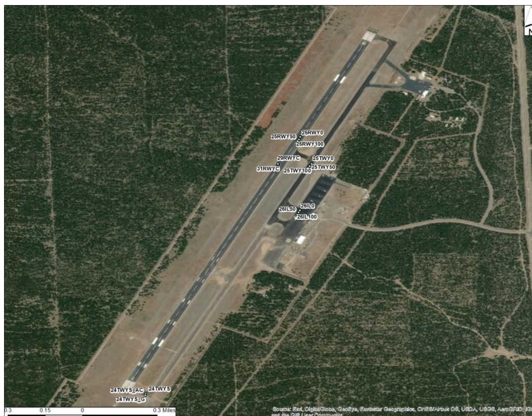
Figure 1. Montana LWD test points plotted on summer imagery that shows pavement surfaces at West Yellowstone Airport, Montana.
