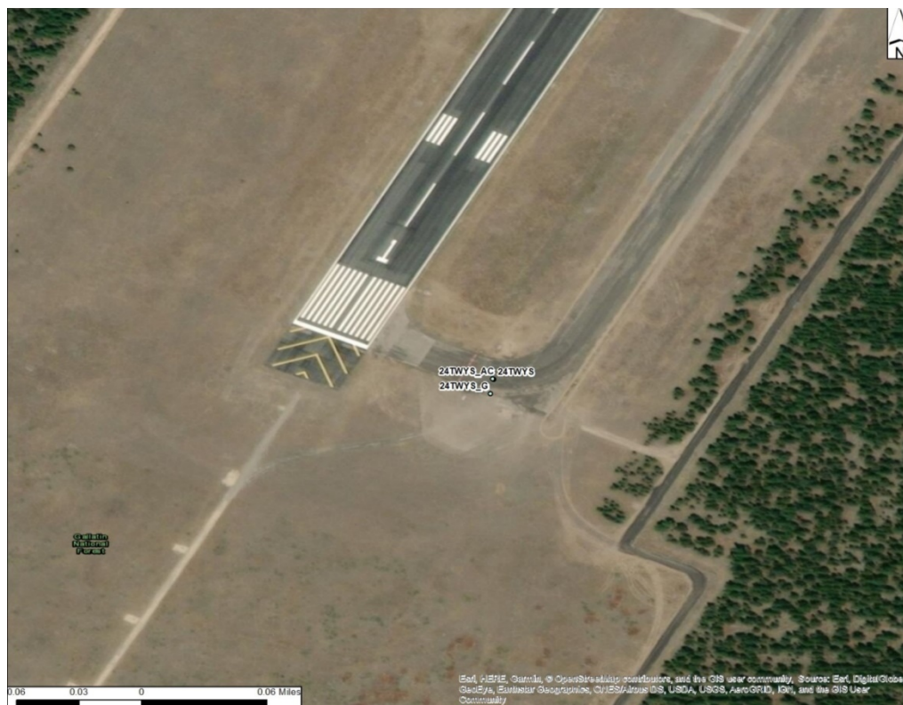
Figure A-2. West Yellowstone Airport south taxiway LWD test points as they relate to the airport pavement surfaces.
