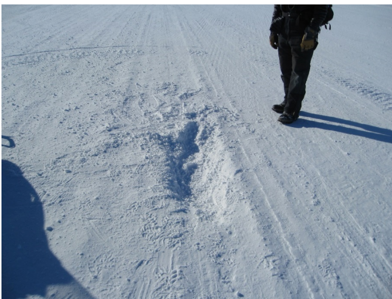
Figure 68. One of a handful of areas showing rutting of the runway surface with the passing of aircraft tires.
