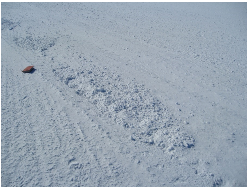
Figure 67. Area showing slight disaggregation of the surface with the passing of aircraft tires.
