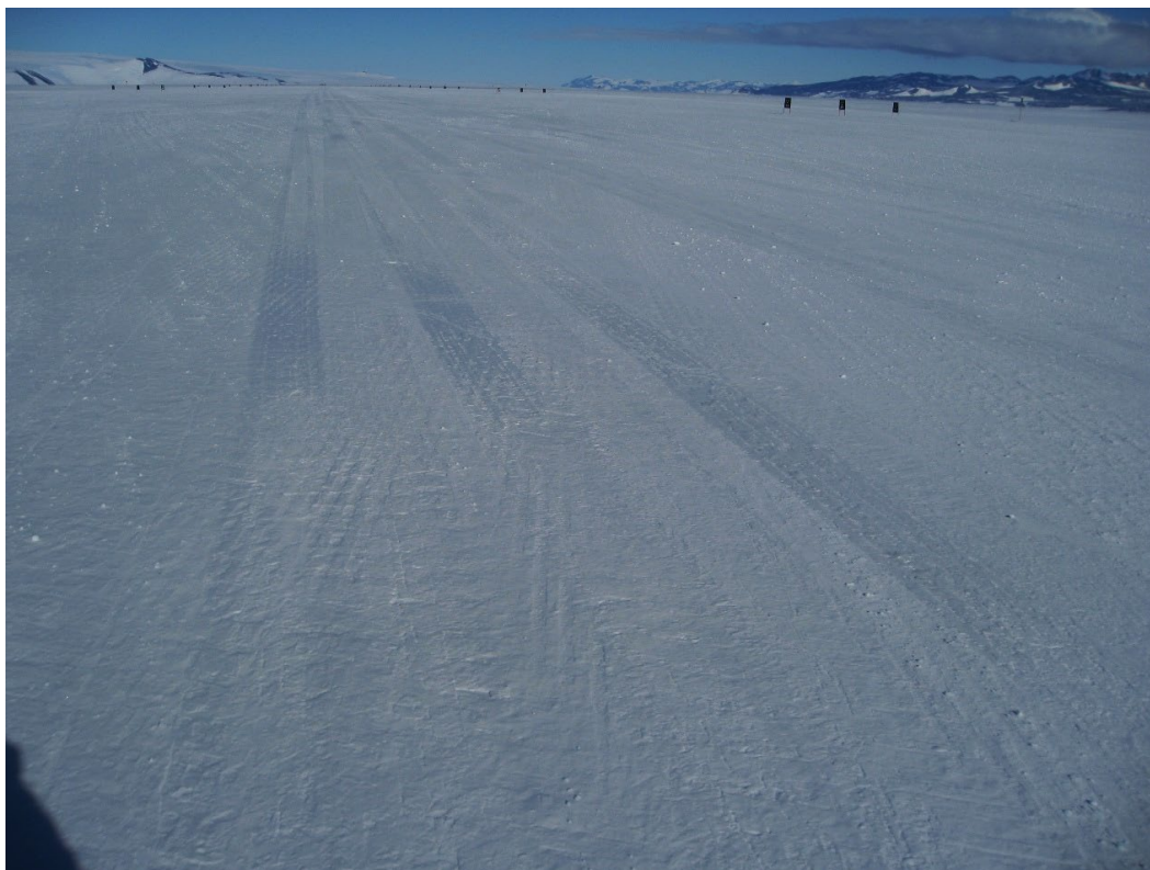
Figure 72. Segments of the main landing-gear tire tracks showing snow-pavement polishing where the main landing gear's antilock braking system created tire slip and segments where tires were rotating without slip in between antilock braking system pulses.
