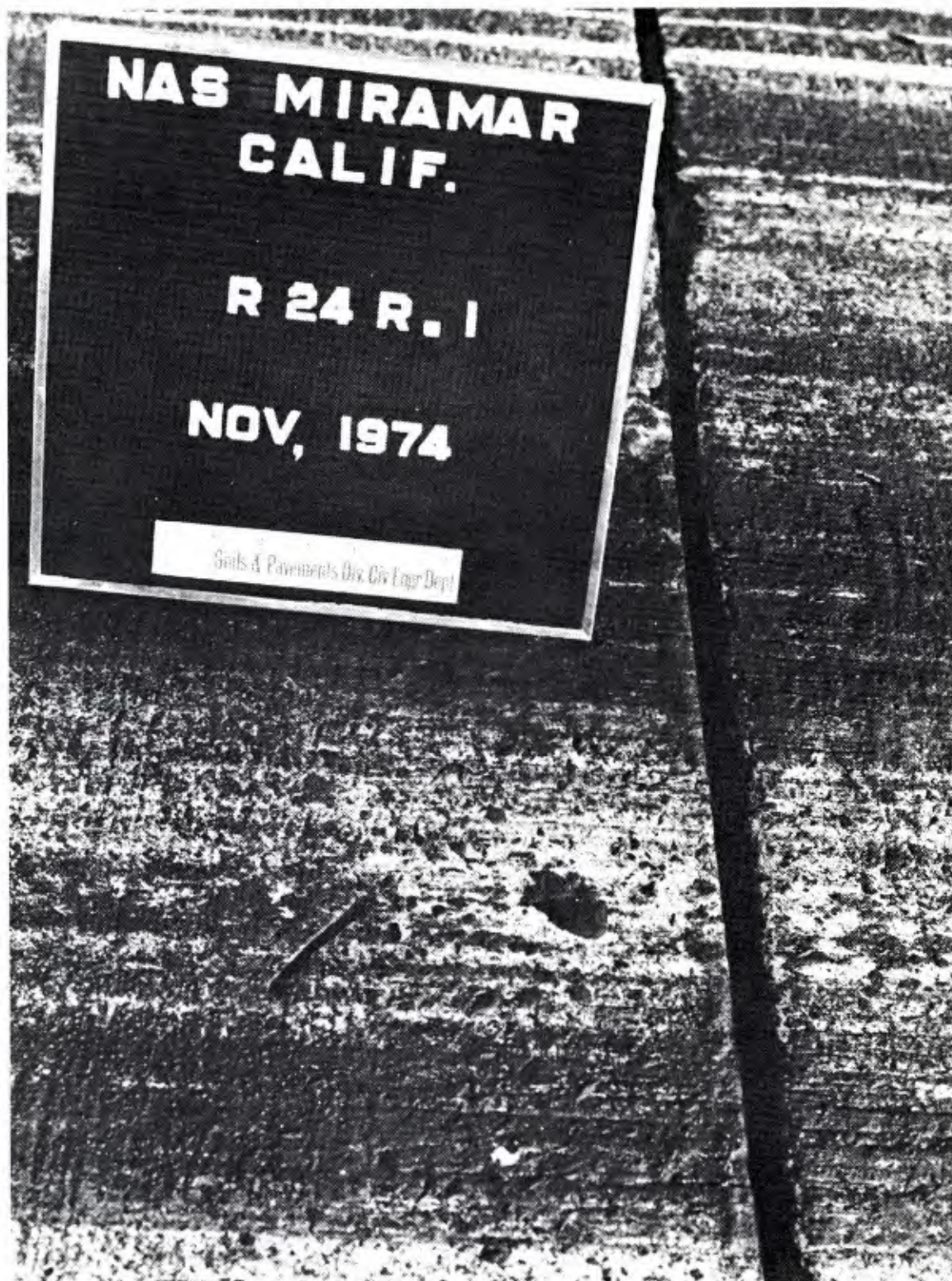
Figure 9. Burned and blown joint seal, Discrete Area R24R-1.
