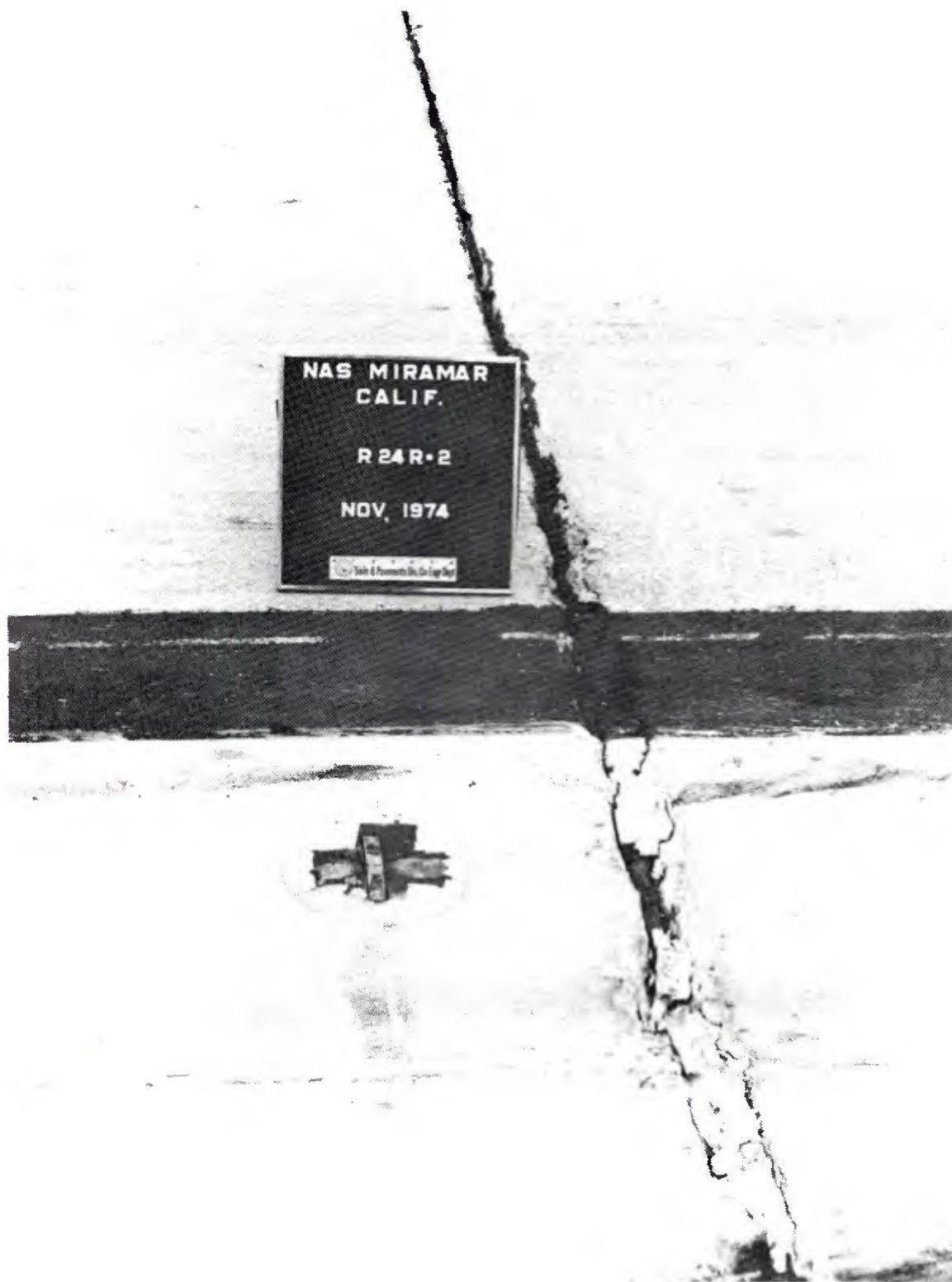
Figure 10. Hardened and shriveled joint seal, Discrete Area R24R-2.
