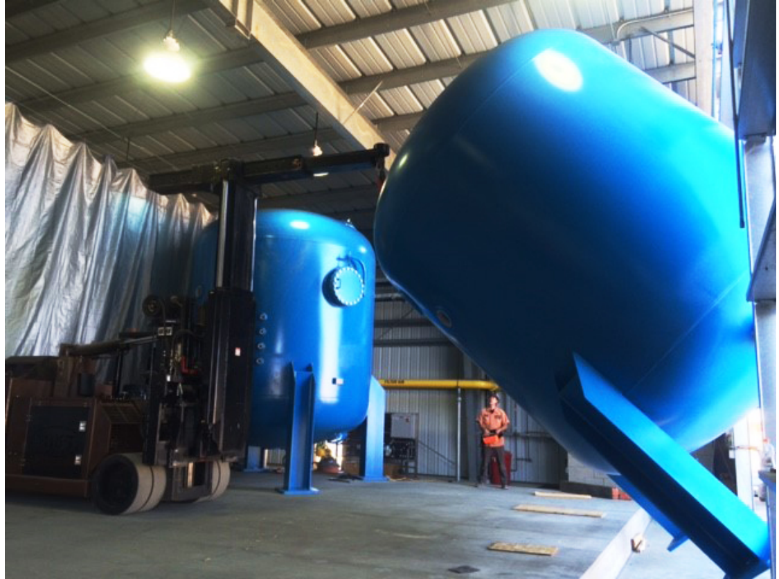
Figure 11 Installation of the FXB Vessels
