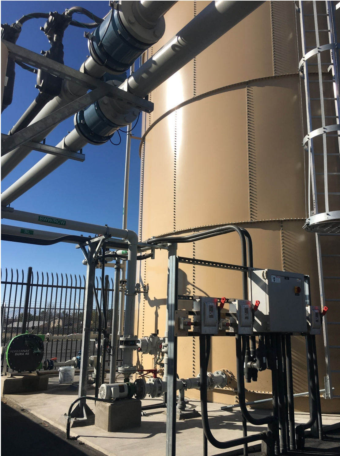
Figure 8 Completed Backwash Waste Tank
