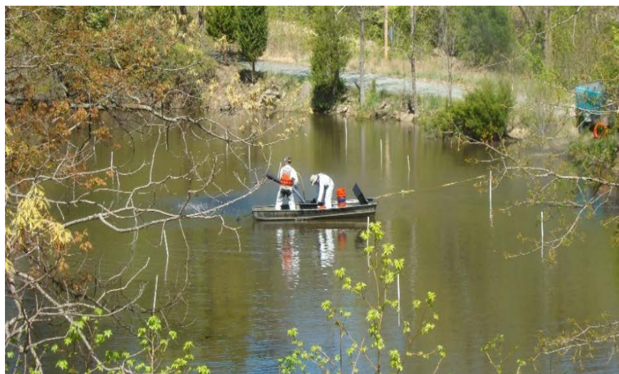
Figure 39. Application of Amendment with a VHI from a Flat Bottom Boat.
