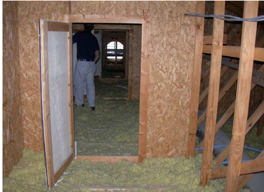
Figure 16. Attic Center Line looking North
