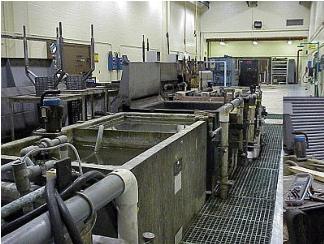
Figure 5-1. nCoP Dem/Val plating line location in Building 794 at FRCSE.
