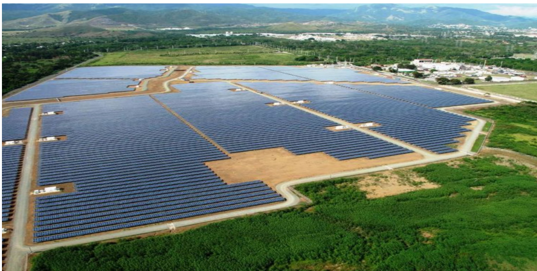
Figure 12. A Solar Array in Puerto Rico prior to Its Destruction by Hurricane Maria in 2017 119
