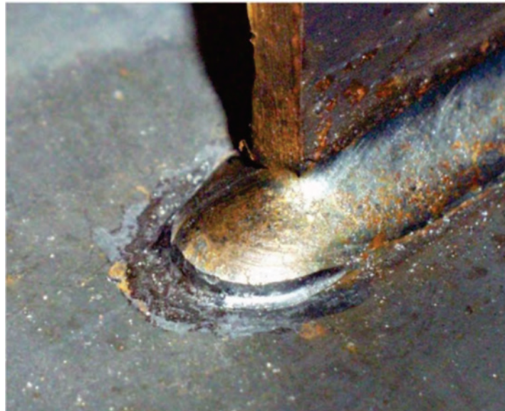
Figure 10. Air hammer peening for repairing fatigue cracks (Dexter and Ocel 2013).
