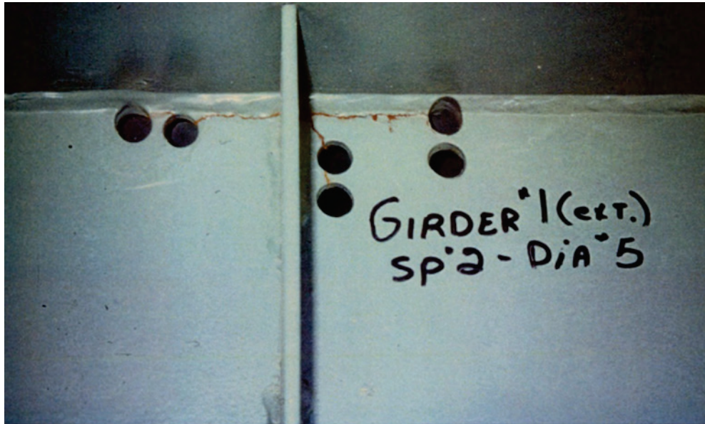
Figure 11. Hole drilling method to stop crack propagation (Dexter and Ocel 2013).
