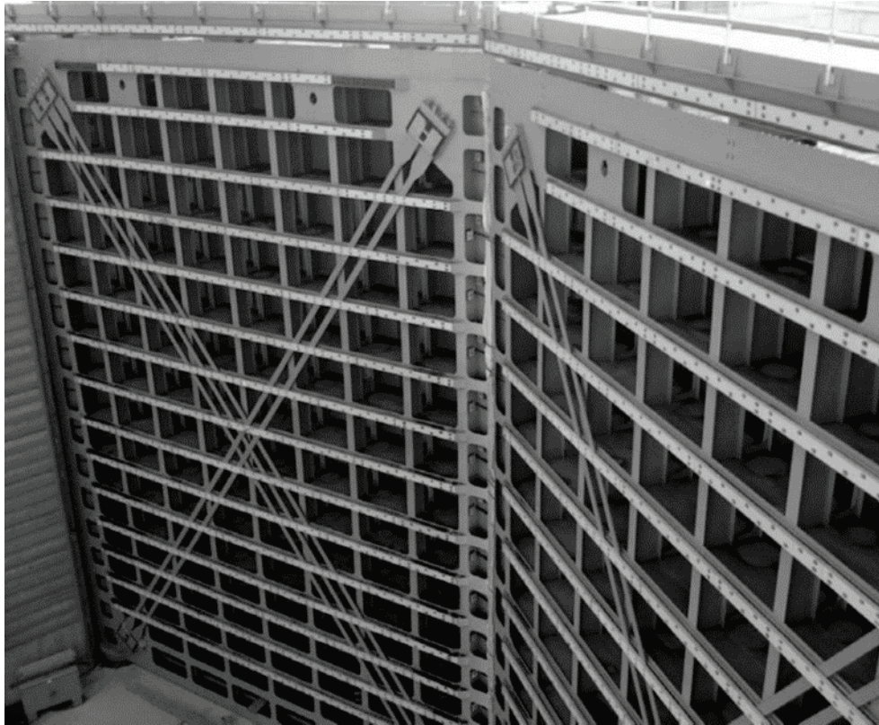
Figure 1. Typical horizontally framed miter gate (USACE 2010).
